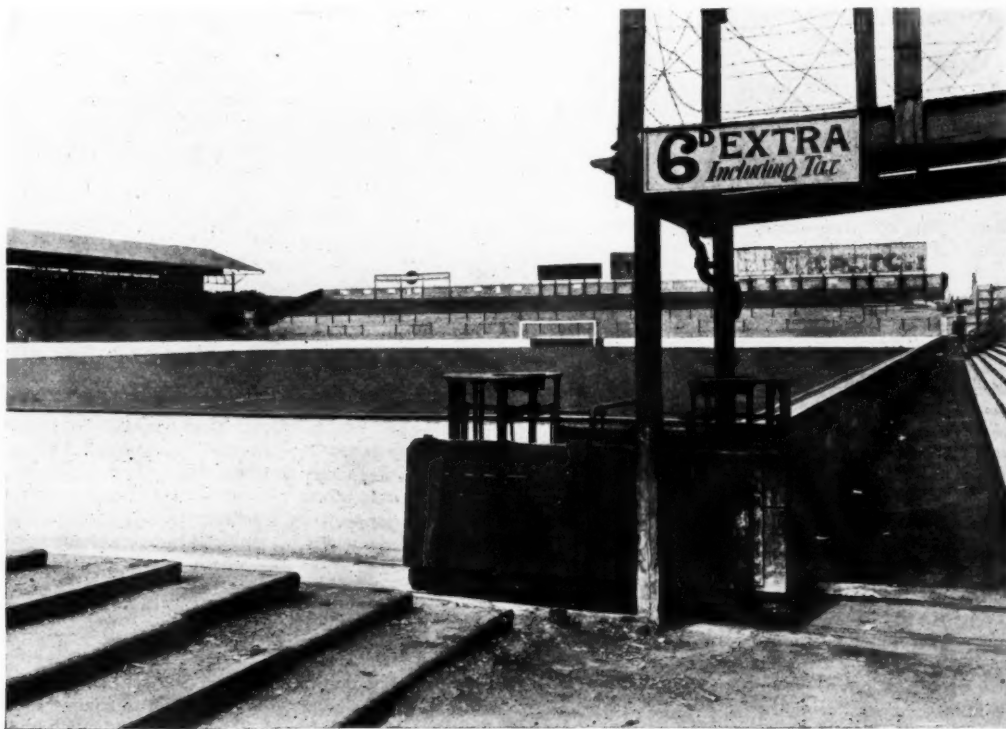
West Ham Football Ground. The reinforced concrete barrier wall round the ground is an unusual feature.
