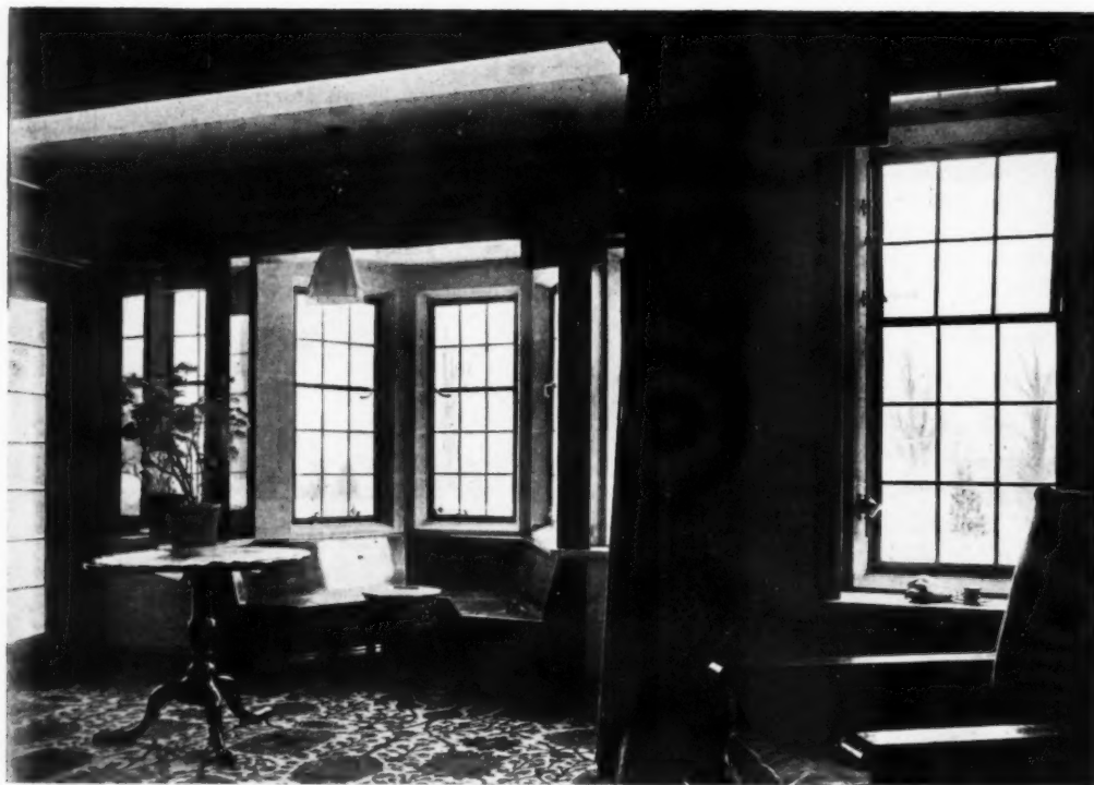
"Warnford": the sitting-room. The stone mullions show themselves in the room, and the window boards are of Hopton Wood stone.
