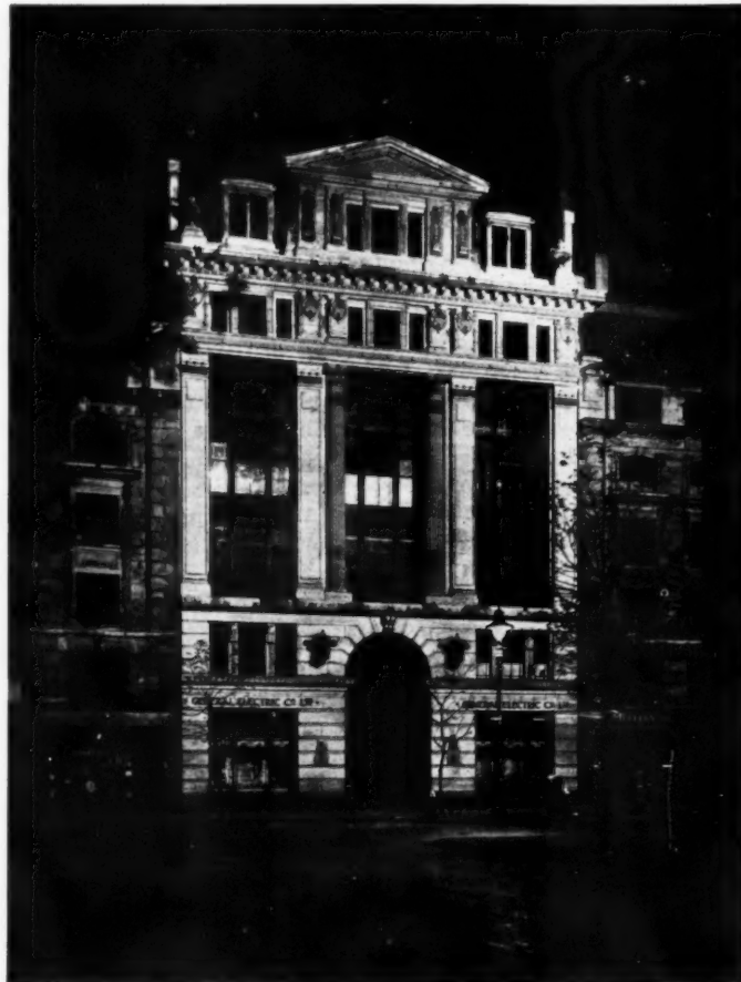
Magnet House, Kingsway. By R. Frank Atkinson.
