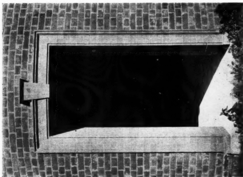
A DOORWAY IN GAUGED BRICKWORK.
