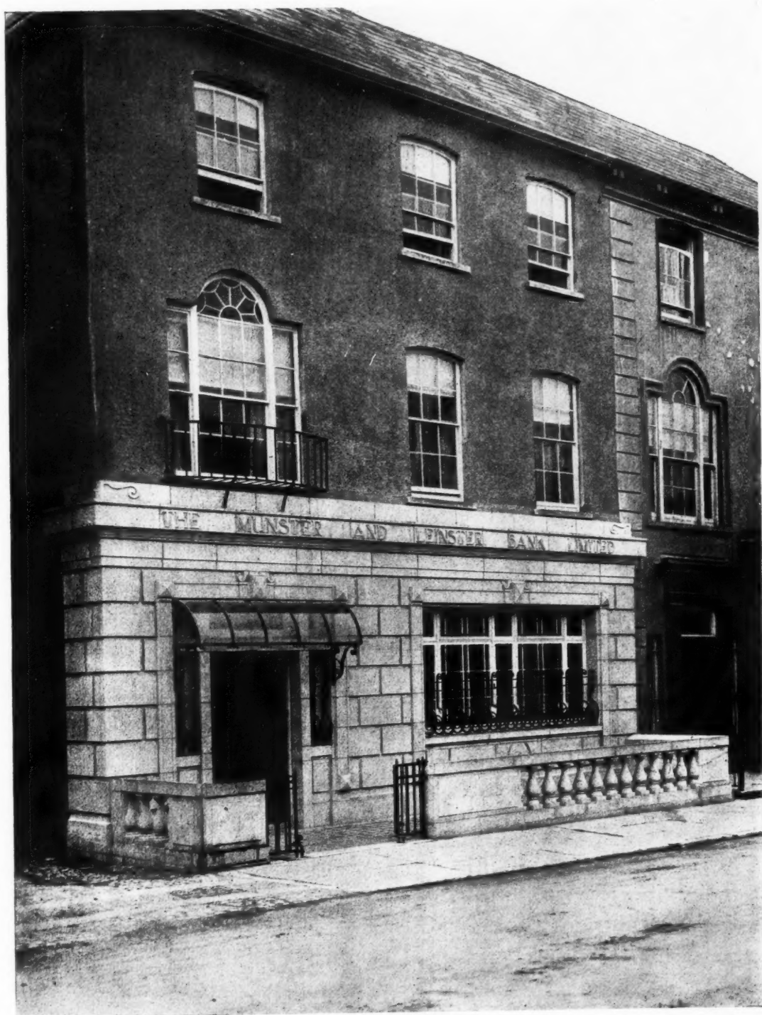
THE MUNSTER AND LEINSTER BANK, MALLOW, CO. CORK. H. H. HILL, B.A., A.R.I.B.A., ARCHITECT.
