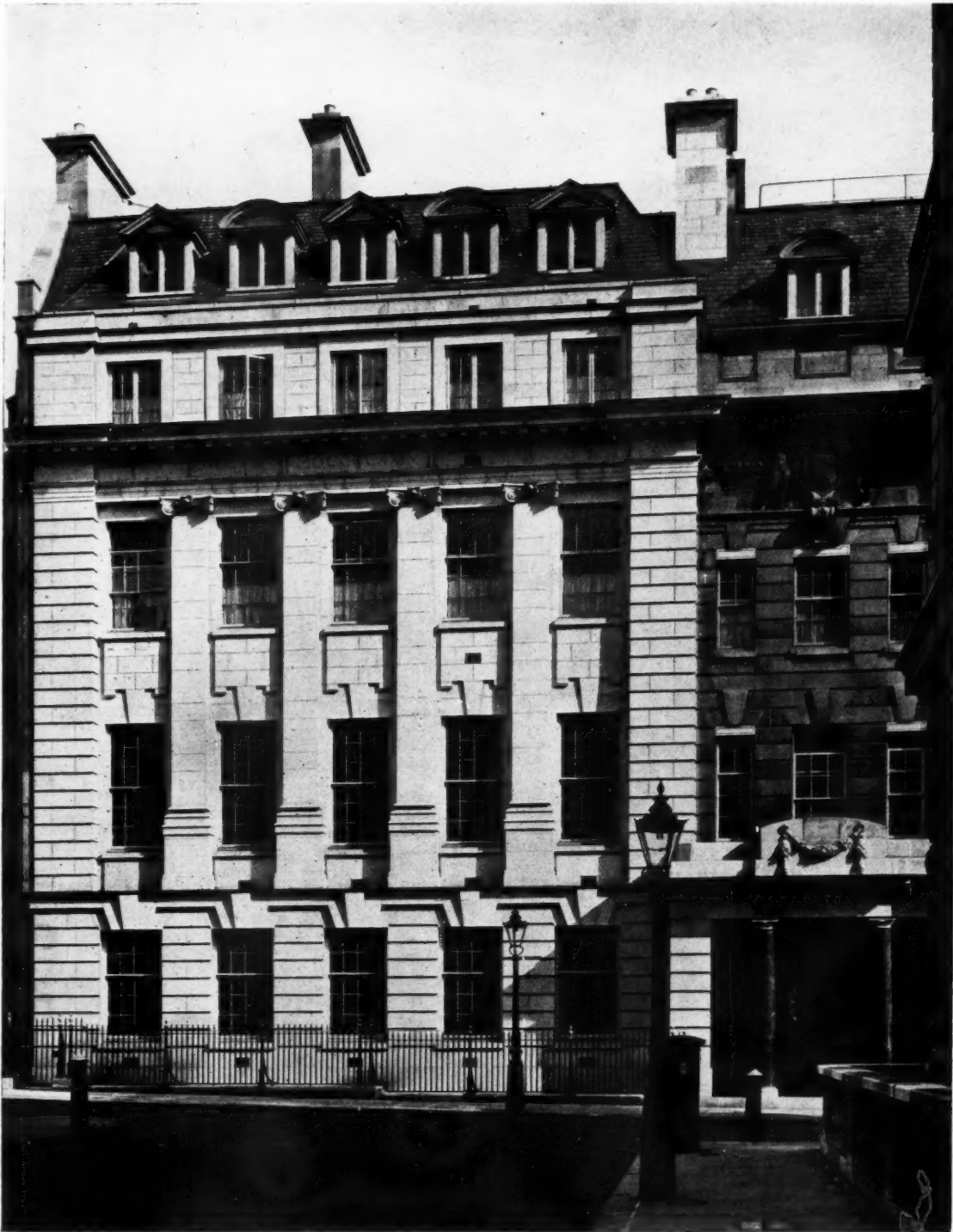
The recent additions to this club follow in detail, as far as possible, those of the original building designed by Sir Reginald Blomfield in 1905.
