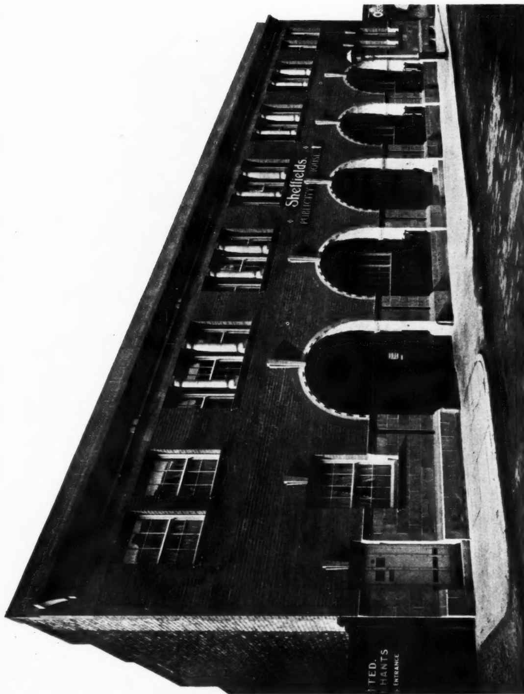
This building is so designed that two more floors may be added at some future time. The structure generally is steel-frame, the walls being of brick, with details in terra-cotta. Further particulars are given on page 514.
