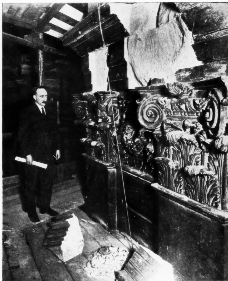
FIG. 5.—THE FRACTURED FRIEZE OF ONE OF THE PIERS.
