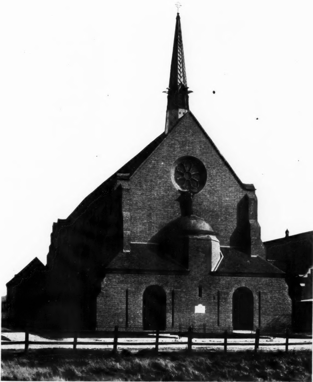
The principal feature of this church is a great nave, with unusually narrow aisles. The small projecting building at the north-east angle is the chapel. The structure is entirely of brick. The fîche is of English oak, and the inner porch doors are covered with hide.
