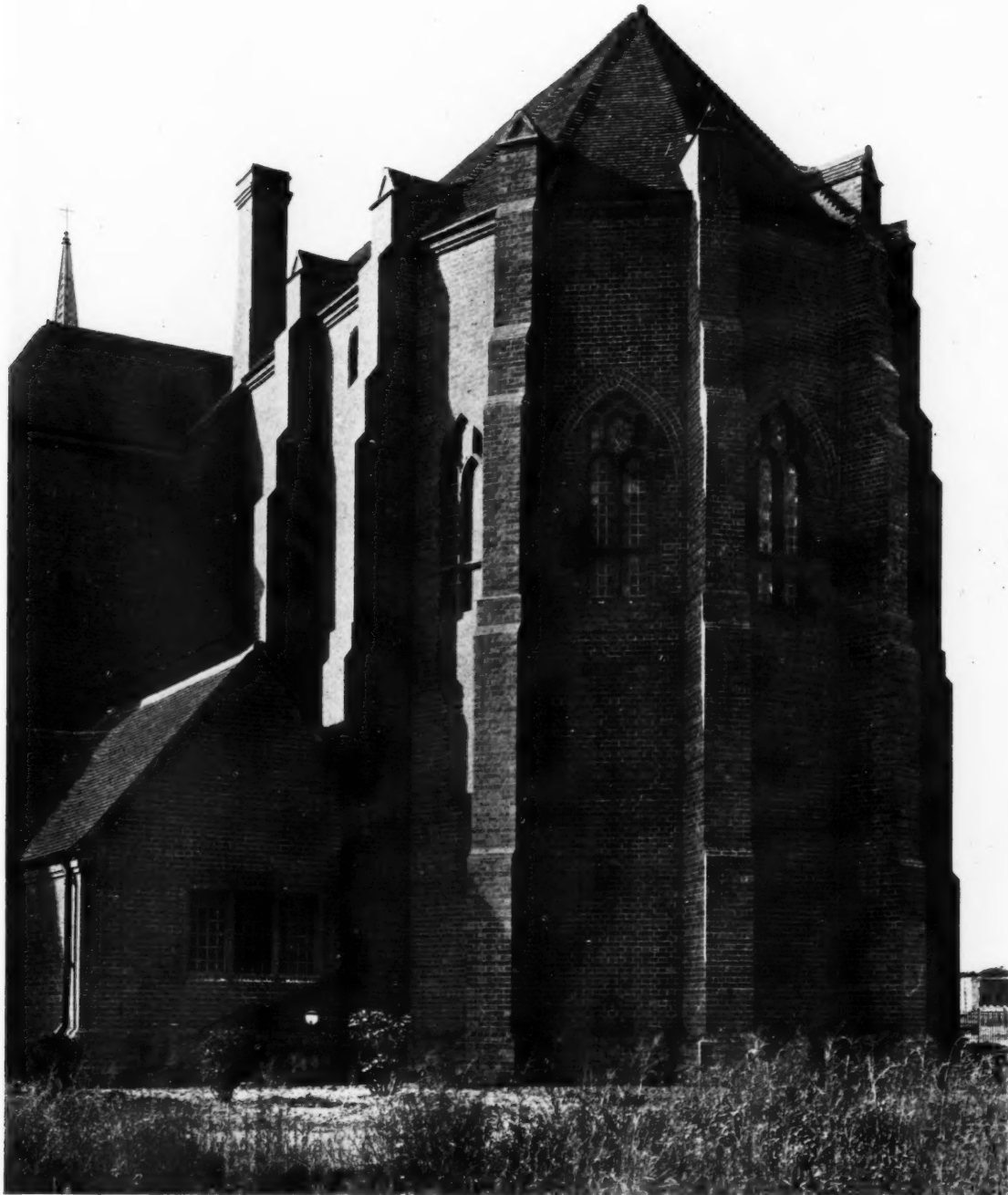
A view of the apse from the south-east. The small projecting building within the angle is the clergy vestry. The fabric is entirely of brick, the roofs being covered with tiles.
