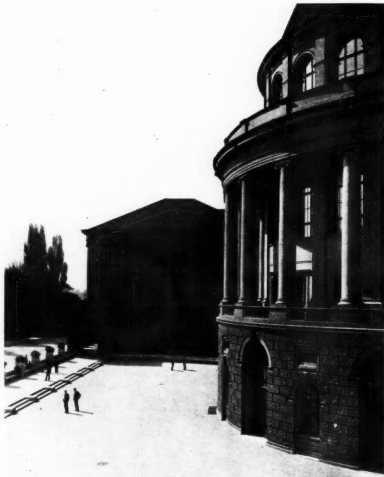
THE FEDERAL TECHNICAL HIGH SCHOOL: THE FRONT COURT.
