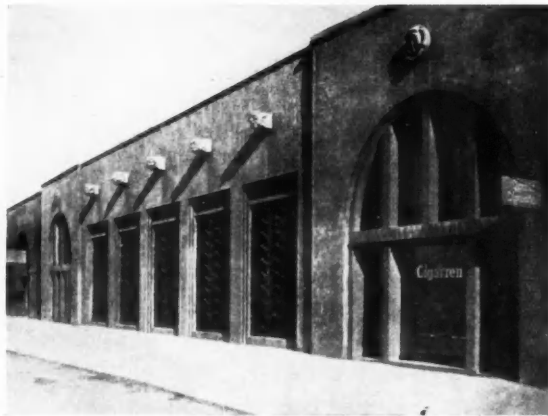
NEW MOTOR WORKS, ESSEN.
