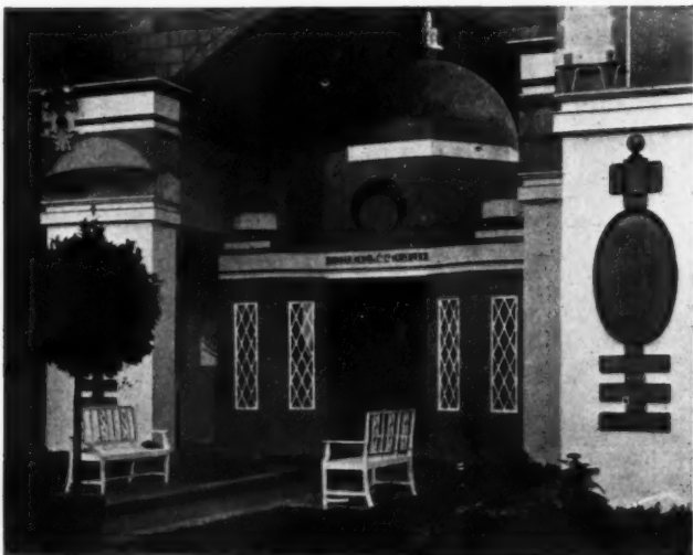
THE BRUNNER-MOND PAVILION. CLOUGH WILLIAMS-ELLIS, ARCHITECT.
