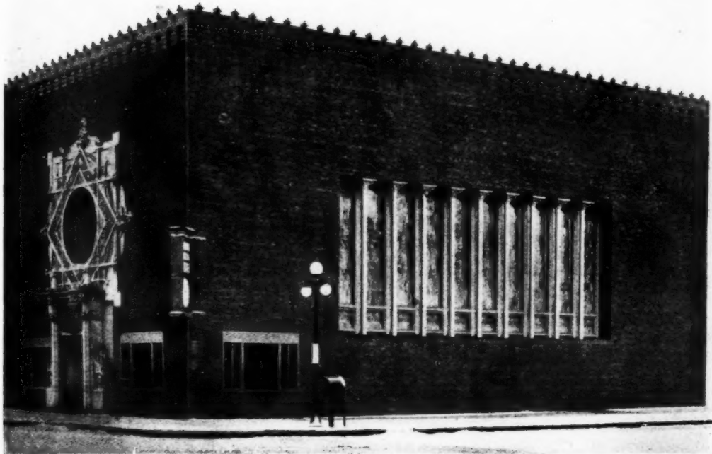
THE MERCHANTS' NATIONAL BANK, GRINNELL, IOWA. THE LATE LOUIS H. SULLIVAN, ARCHITECT.
