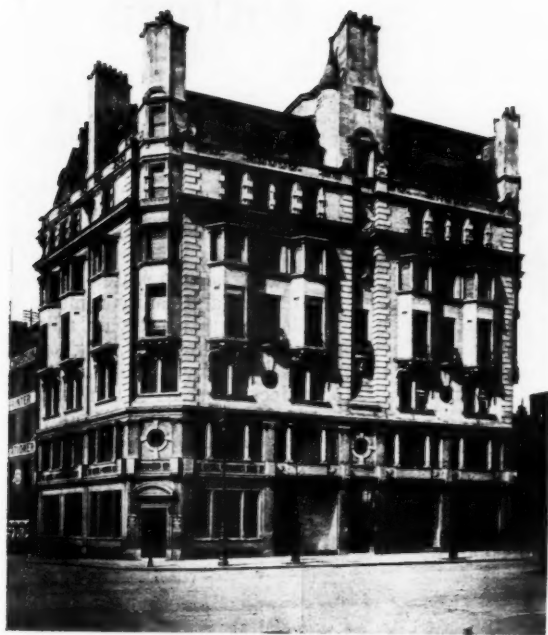
ANOTHER EXAMPLE OF TOO CONSPICUOUS CHIMNEYS.
