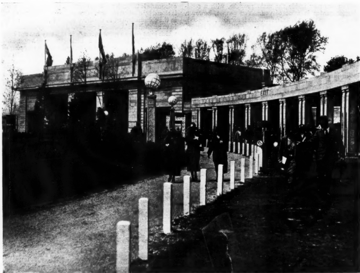
THE NORTH ENTRANCE, WITH ITS SEMI-CIRCULAR COLONNADE. SIMPSON AND AYRTON, P.P. AND F.R.I.B.A., ARCHITECTS.
