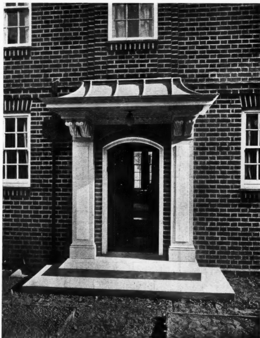
A DETAIL OF THE ENTRANCE DOORWAY.
