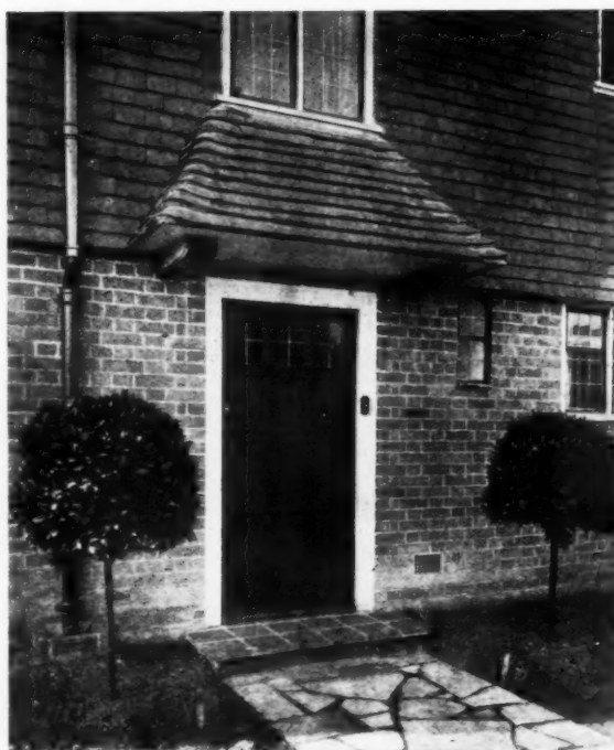
A DETAIL OF THE DOORWAY.
