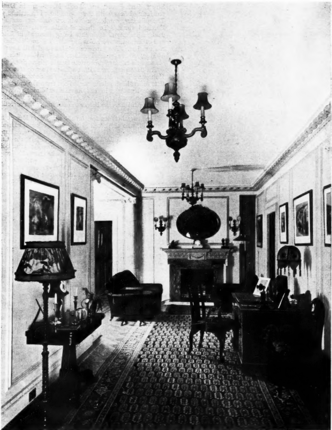
NEW RESIDENTIAL FLATS IN PARK STREET AND UPPER BROOK STREET, LONDON, W.: A TYPICAL HALL WIMPERIS AND SIMPSON, F.R.I.B.A., ARCHITECTS.
