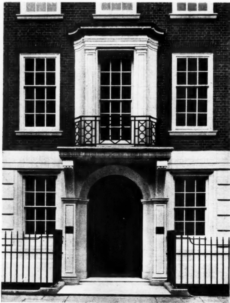
A DETAIL OF THE PRINCIPAL ENTRANCE.
