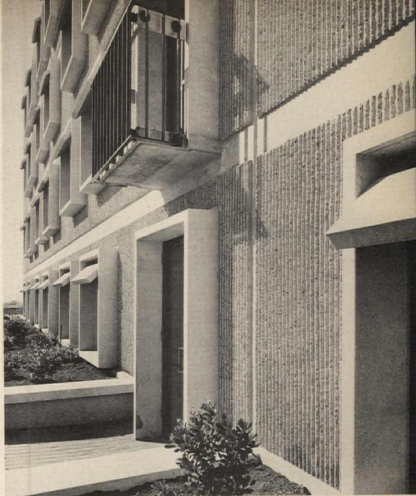
Alta Bates Hospital, Oakland, California, combines reeded and hammered finish on cast-in-place walls. Flat surfaces are lightly abrasive blasted, window units acid etched. Rex Whitaker Allen & Associates.
