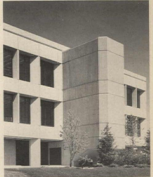
Kemper Insurance Office Building, Low Grove, Illinois, shows light abrasive blasted, combination precast and cast in place concrete (above). Welton Becket & Associates.
