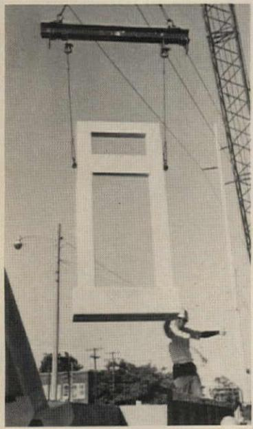
The 6'-6" x 14' window units are composed of five pieces of Shadow Vein Limestone bonded together.
