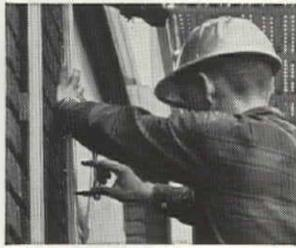
Vertical struts are anchored to existing facade.
