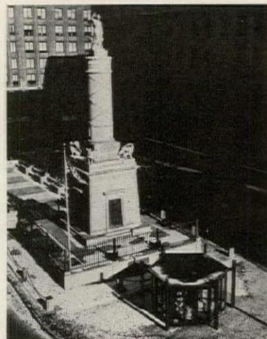
**Hexagon on the Square:** The rigid steel structure has a matte bronze-tone finish on the roof, adjustable display shelves and wooden storage bins—and even radiant heating for Baltimore's cold months.
