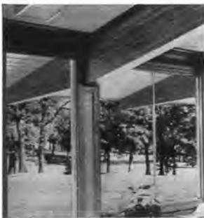
Cantilevered glulam beams extend the roof to form a canopy which protects the window areas from the sun. Classrooms receive natural light from three sides.
