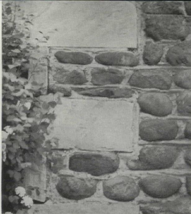
FIG. 2. A MASONRY WALL OF THE FIRST HALF OF THE EARLY PERIOD BUILT UP OF FIELDSTONES OF VARIOUS SHAPES, SIZES AND COLORS.
