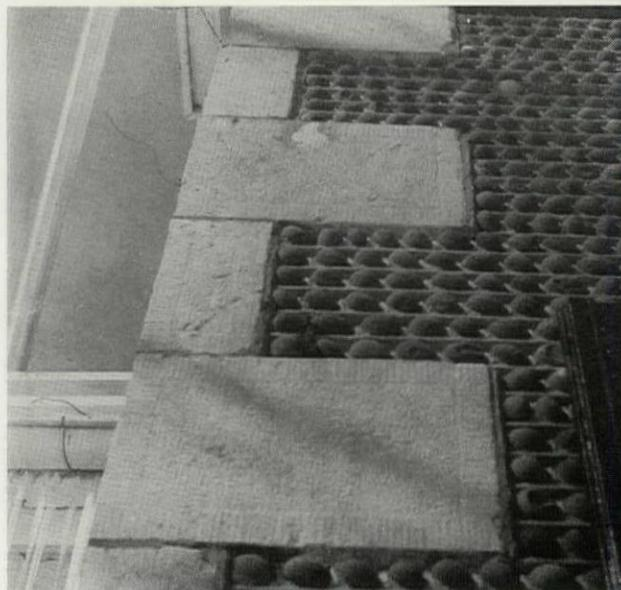
FIG. 6. LAKE-WASHED STONES OF THE LATE PERIOD, CAREFULLY SELECTED FOR COLOR. NOTE THE PROJECTION OF THE COBBLESTONES, AND THE TOOLING OF THE QUOINS.
