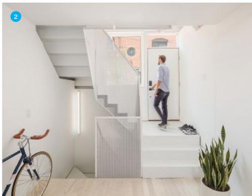
**1.** A custom metal stair by En-Motion Designs connects the floors at the front of the house; perforated metal baluster panels ensure that daylight from the front windows is still able to enter the living spaces. **2.** Gypsum board walls and ceilings in the main entry and throughout are coated in Sherwin-Williams paint, and are complemented by light Bellawood floors.
