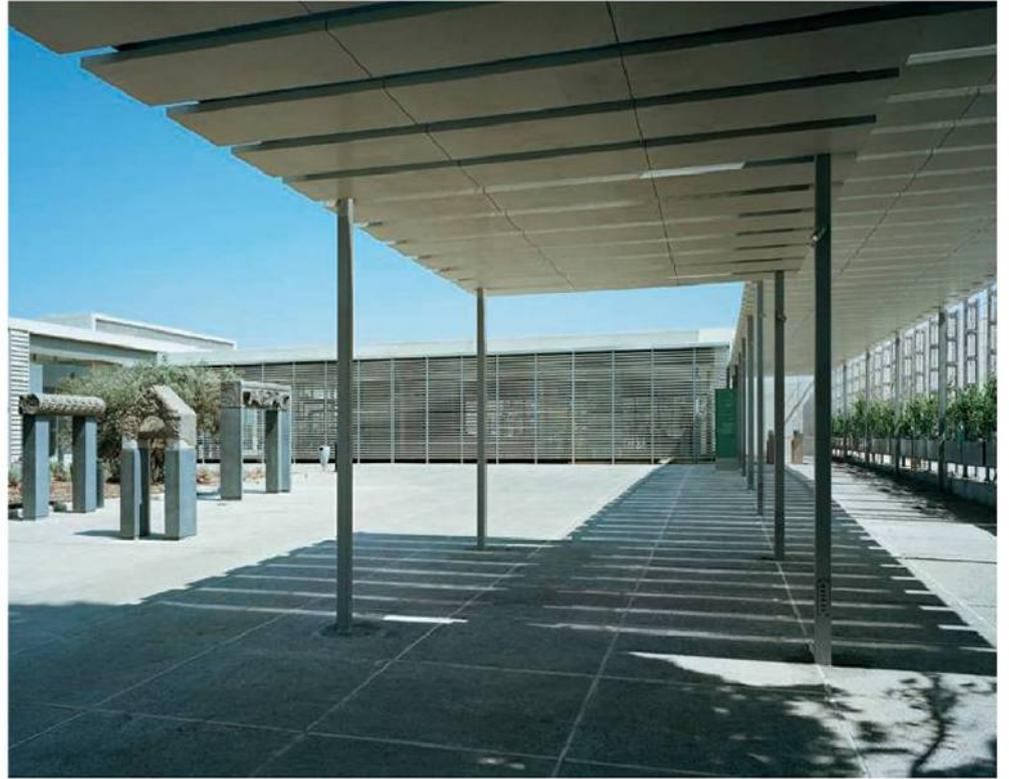
The design team tested the light-reflecting capabilities of different louver shapes to find the best forms for maximizing diffused natural illumination, depending on whether the louvers were for the new structures' north-south façades (right and above) or east-west ones (above). Below, a study of the louver design for east-west façades.
