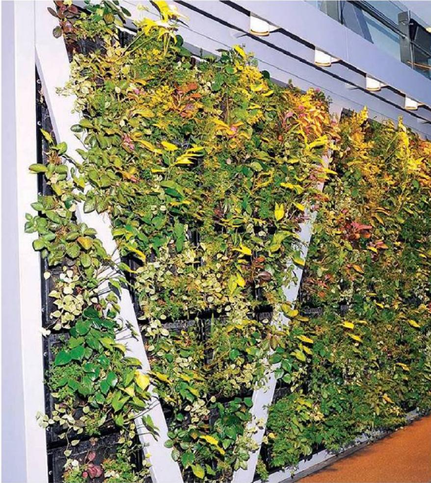
Elmich green walls utilize a **Vertical Greening Module (VGM)**, which is assembled from high-strength lightweight plastic. Modules are 20" by 22" and up to 10" deep. Each VGM contains a geotextile liner placed in a mostly inorganic planting mix. The living walls reduce sound transmission, enhance air quality, and reduce stormwater runoff. • [elmich.com](http://elmich.com) • Circle 101
