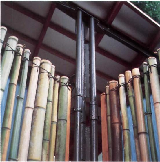
RIGGA designed and built lyrical garden pavilion in Portland (these pages). Panels made of bamboo poles (above) and translucent fabric sheets pivot open and shut. Unpolished yet carefully assembled components such as steel columns (below), slatted wooden walls (top), and aluminum roof reflect RIGGA's simple, hands-on approach to craft.
