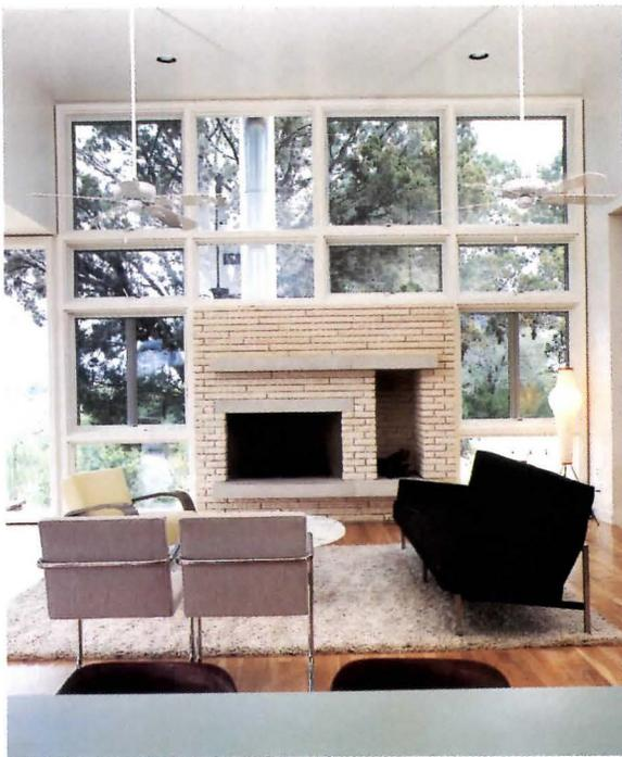
Roof joists that span deck (right) rest on C-channels welded to lally columns and braced by tension cables anchored in wood frame above joists. Deck is structurally independent of enclosed spaces. Glazing (top) is composite of fixed glass and commercially produced operable windows installed in wood frame. Living room fireplace (above) occupies 14-foot-tall space that reflects Alter's interest in postwar modernism.
