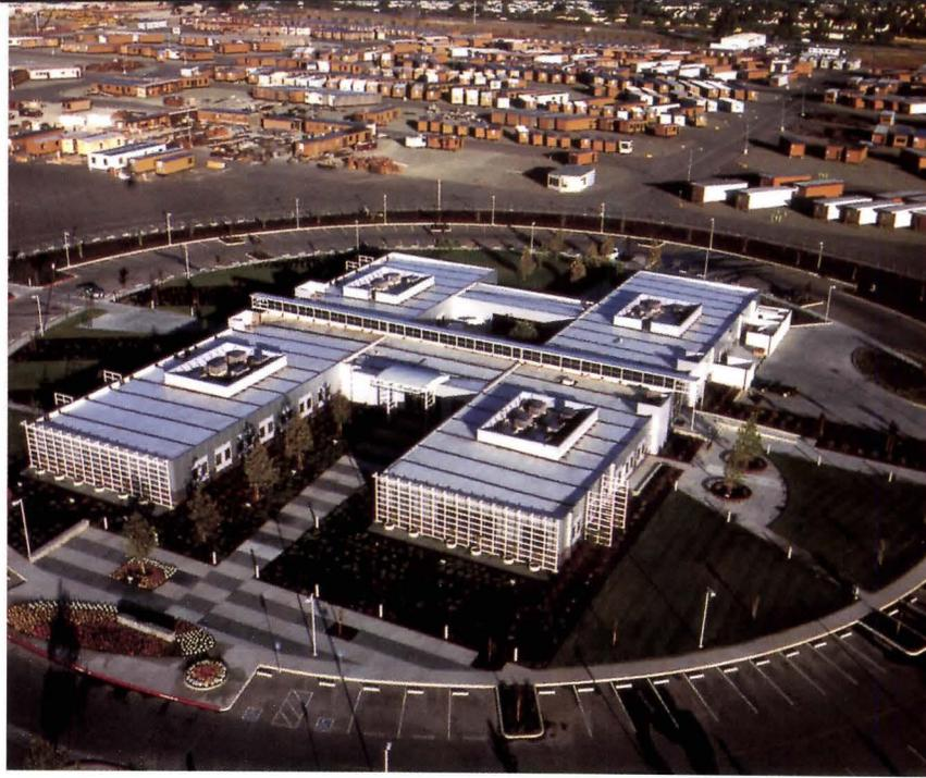
McGrath Rentcorp headquarters in Livermore, California, (above right, facing page) is constructed of 12-by-60 foot **modules** docked along central organizational spine. All units were **lifted by crane** (below) onto poured-in-place concrete foundation and bolted together in four days.
