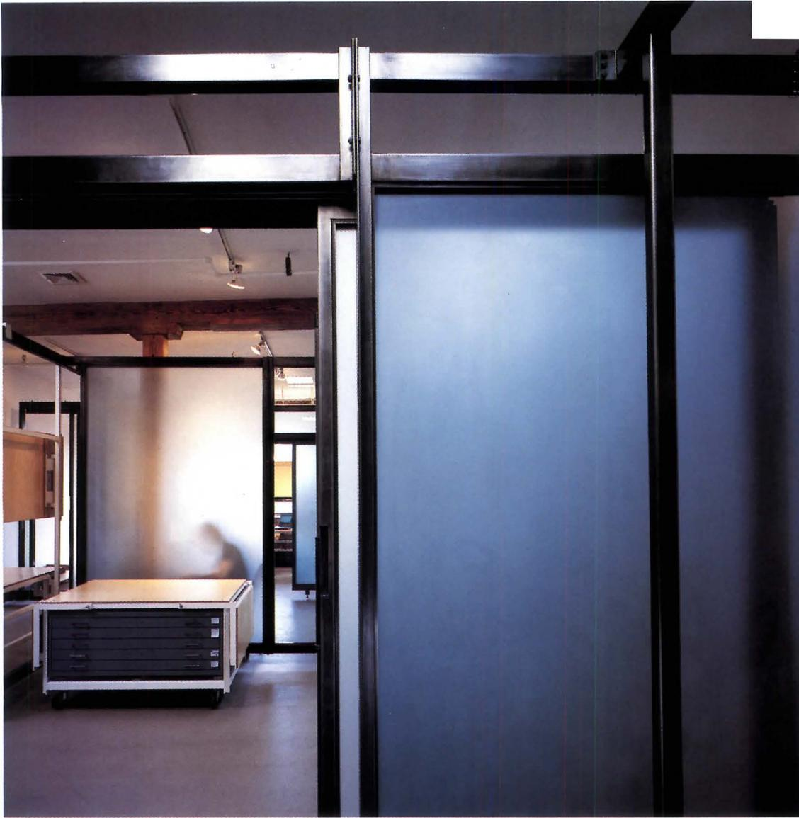
FACE delineated photographer's 1,800-square-foot studio with "spatial equipment"—freestanding steel-and-glass partitions on levelers (above) and steel desk (below left). Detachable storage units and workstations (facing page bottom) are suspended from steel framing system. Translucent sand-blasted glass (below right) diffuses light that enters through large skylights and south-facing windows (facing page top), which creates atmospheric shifts in space throughout day.
