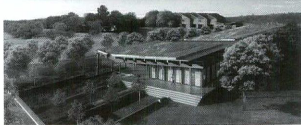
Architect: HKS Architects, Richmond; Thompson & Litton, Wise Project: VCU Dental Clinic, Wise County
