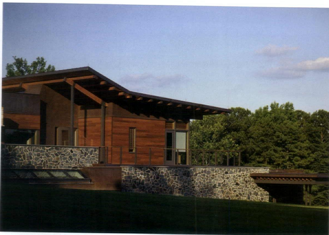
The greenstone of the original façade (above) follows along that of the extension too, meeting the rich red of Spanish cedar. People in windowless offices at the second, or "Earth," level benefit from indirect natural light (below), via windowed roof areas facing north.
