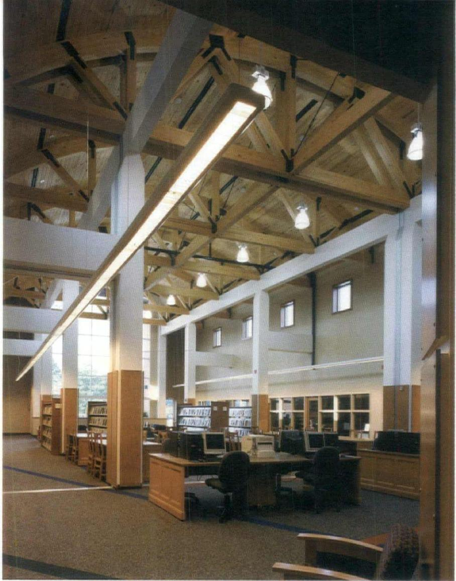
Second-floor spaces reside beneath a towering vaulted ceiling supported by stout wood-and-steel bowstring trusses.
