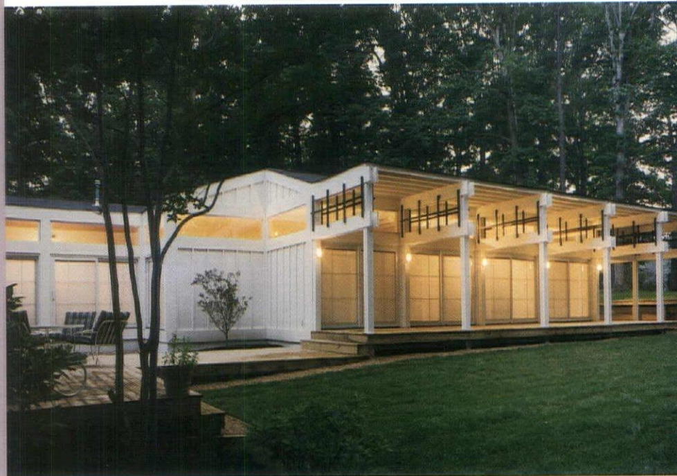
Oversize beams, tied together by a contrasting web of 2"-by-2" wood elements, produces a light feeling on the veranda enclosure (above). The open ceiling lends a spaciousness to the interior (below left).
