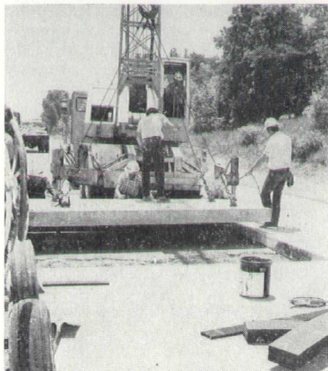
Precast Concrete Patch is placed on Interstate Rte. 95.
