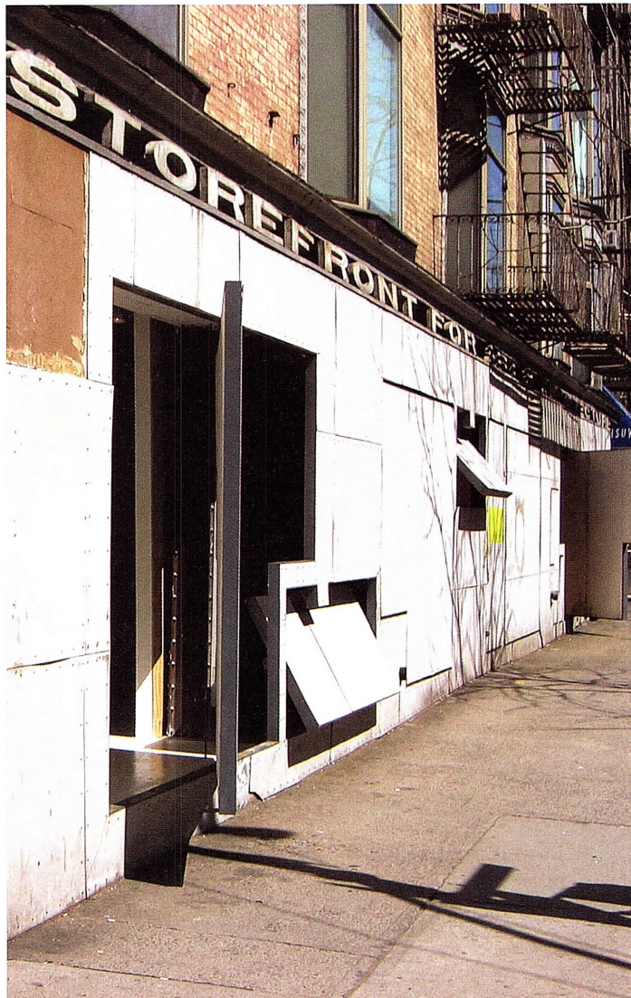
The Storefront’s storefront has a number of cutouts that pivot open (top) The façade is in much need of repair (bottom)
