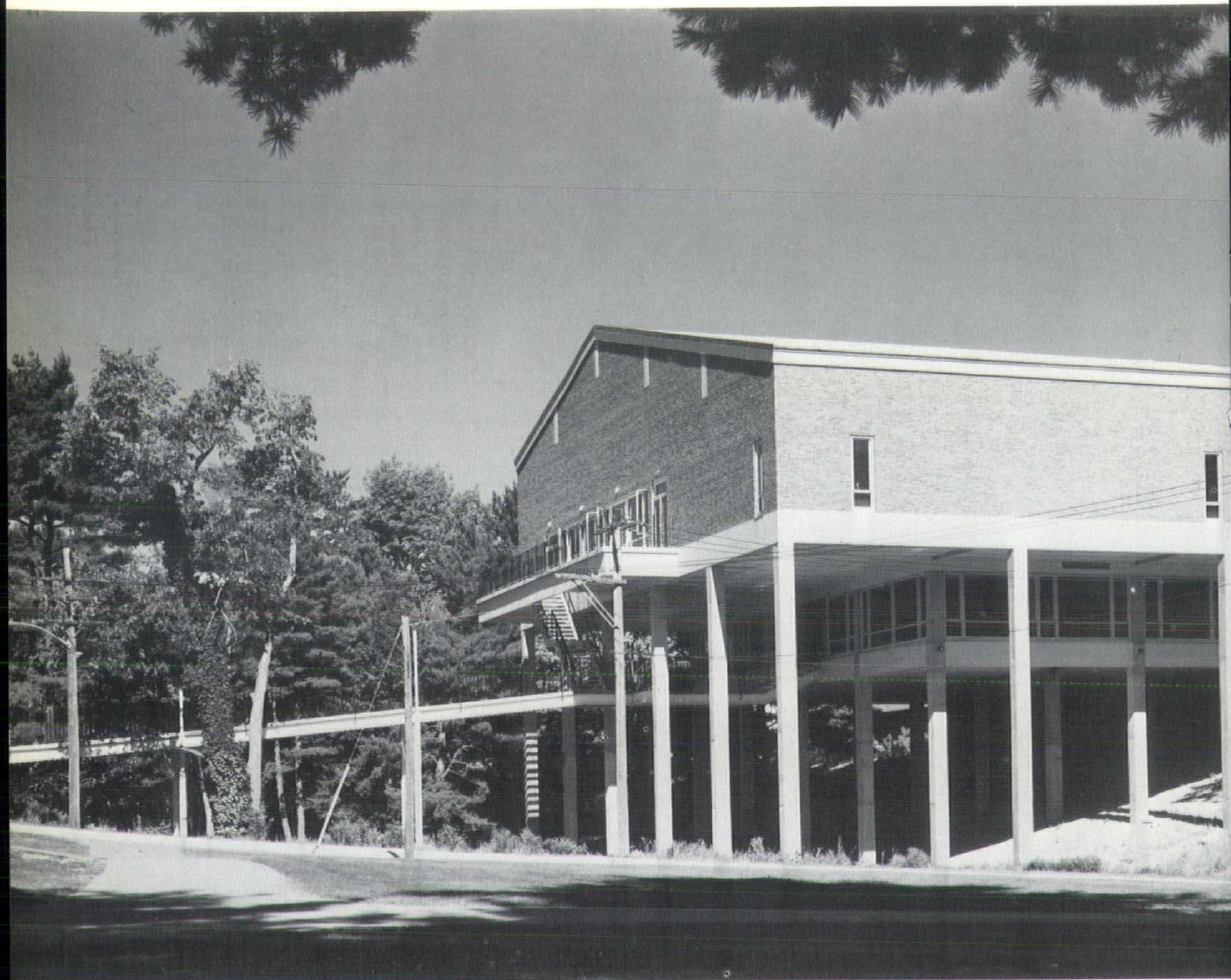
The addition, opened in September, viewed from the East; Devine Hall is just off camera, left. The bridge is steel-framed, and 80 feet long, soaring over the ravine. It has timber planking, and connects with the first floor, rear.
