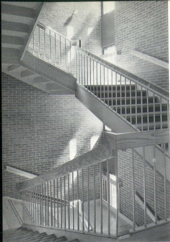
Detail of the east stairwell, connecting the three floors with outdoors. Below, general view, with the addition's south-west corner at left. There are at present no plans to make use of the space under the lower floor. Casement windows were favored.
