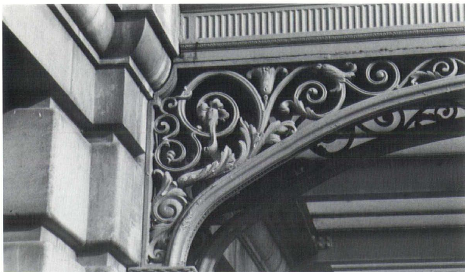
Detail of the wrought-iron work on the entrance to the Burlington Depot.
