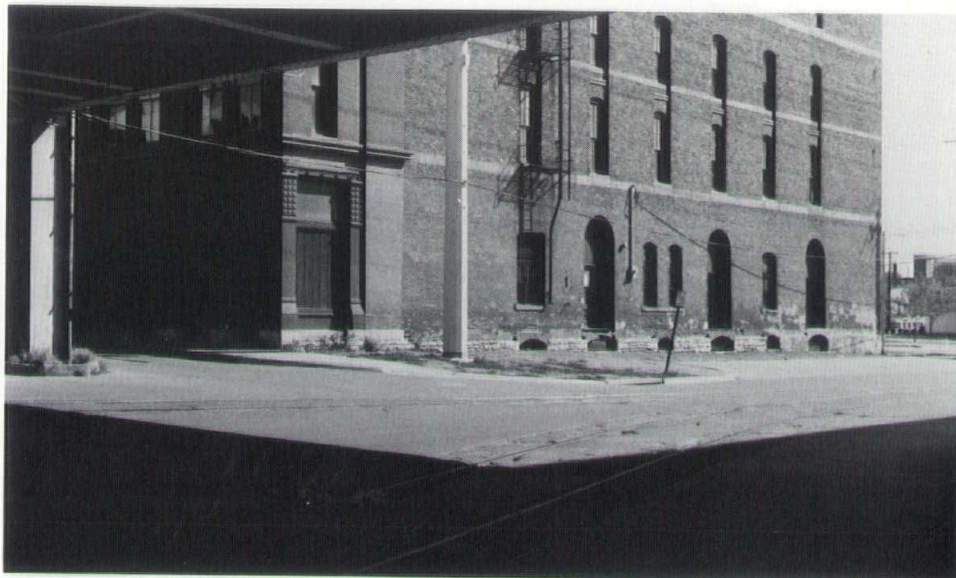
View from the viaduct
