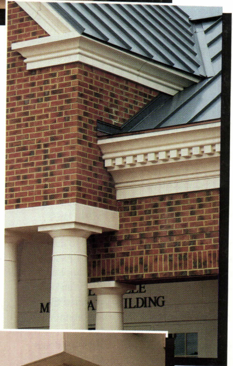
FRP cornice, column covers, Municipal Building, Kenersville, NC
