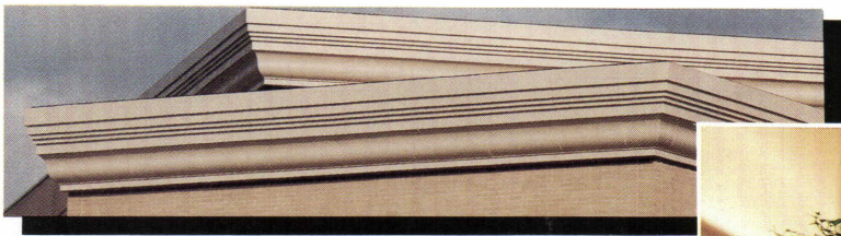
Cornice system, Belk's Department Store, Pineville, NC
