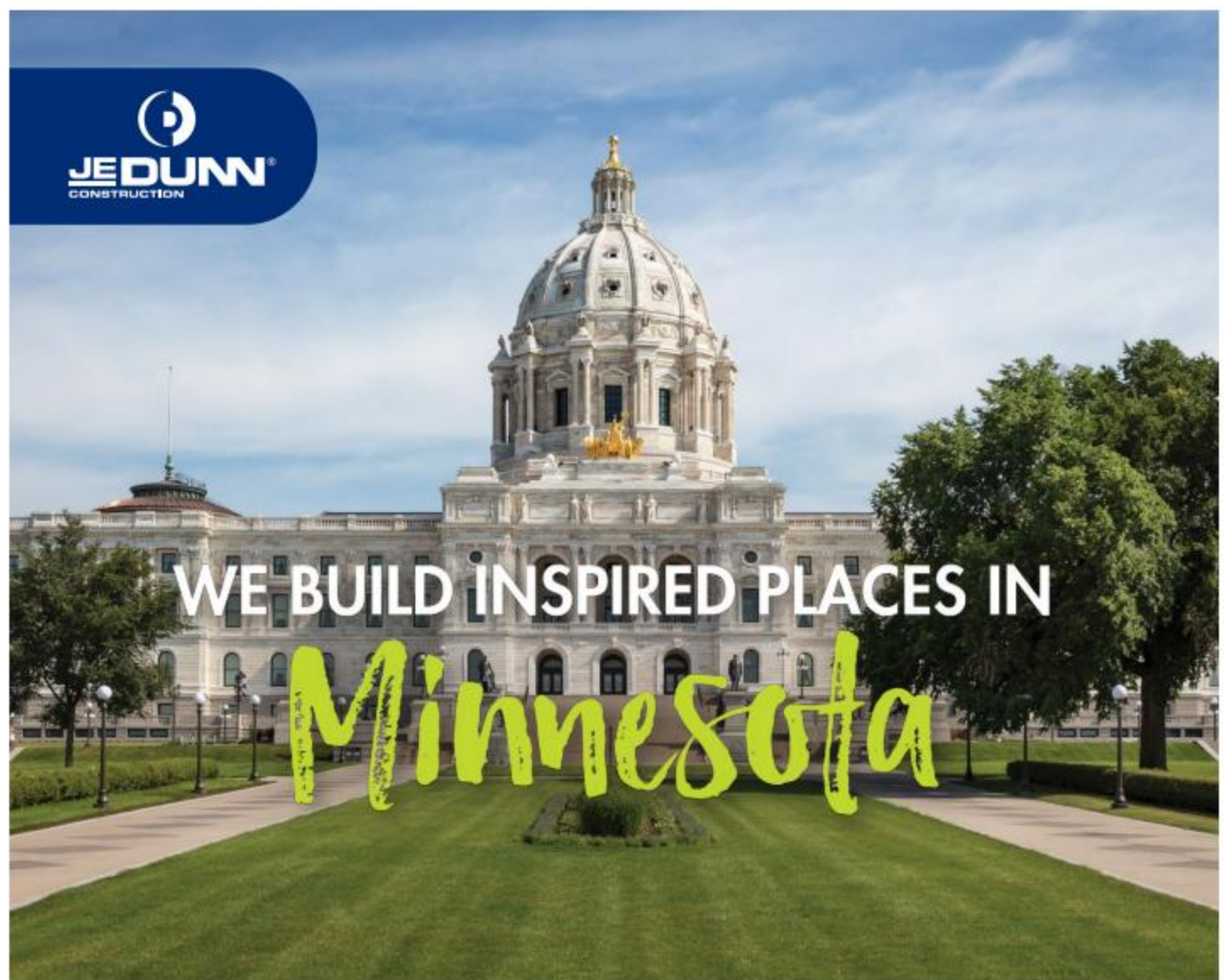
Minnesota State Capitol Restoration HGA
