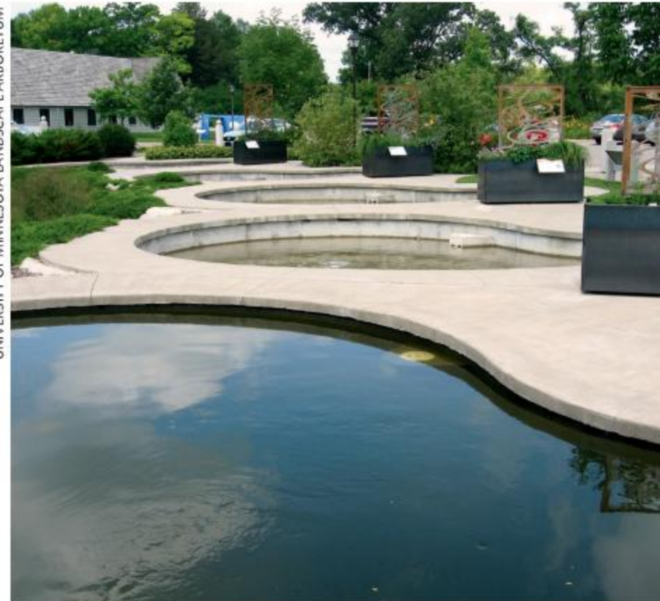
With its five distinct watersheds (raindrop-shaped pools), each with a different permeability, the arboretum's Stormwater Runoff Model Parking Lot allows researchers to study the effects of surfacing on stormwater.
