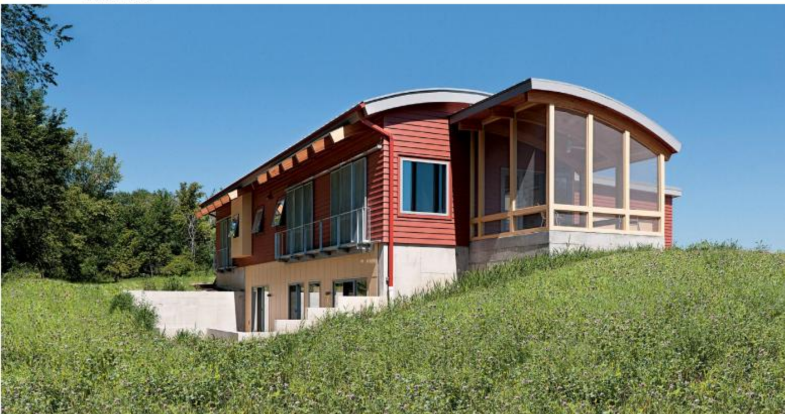
The LEED-Gold Spear House pursued a number of passive and related strategies. The roof overhangs were designed to minimize heat gain and control direct solar gain in summer, and the glazing has a high solar heat gain coefficient (SHGC).
