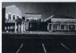
Burnham Brook Center
