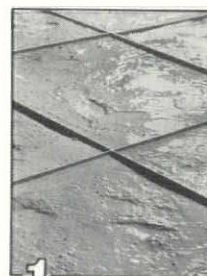
1 TERRAZZO sub-bed divided by plastic strips.
