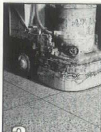
3 Grinding and finishing TERRAZZO floor.
