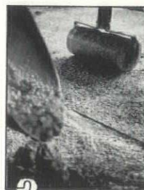
2 Placing and compacting TERRAZZO topping.
