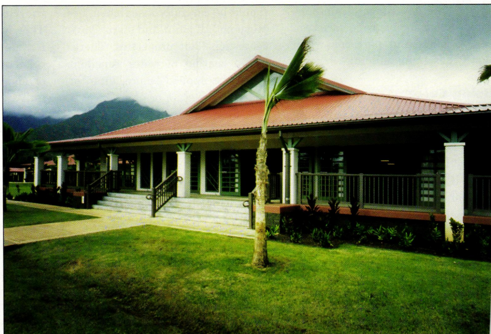
The cafetorium building is equipped with deep lanais which serve as a pre-function area, clerestory windows and security doors.
