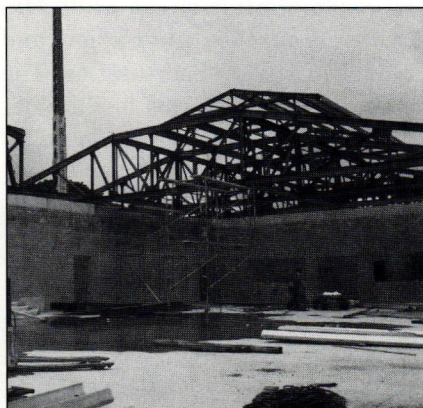
Kea'au High School (under construction)
