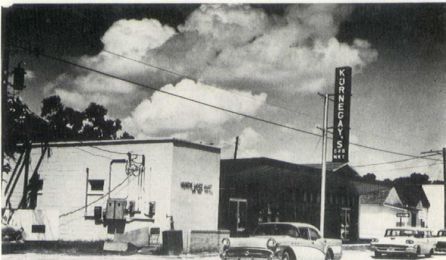
This building occupied by a grocery store and bank was one of the few structures that escaped destruction during the hurricane.
