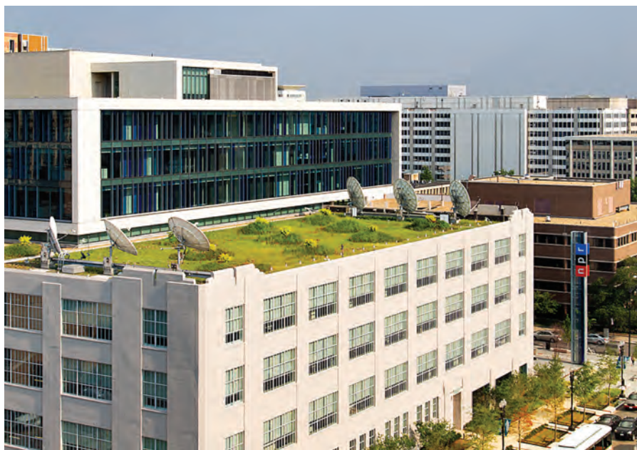
Aerial view of the NPR complex, showing the green roof atop the historic C&P Telephone Company warehouse.
