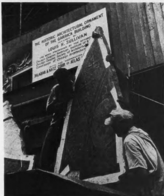
Photo: Commission on Chicago Architectural Landmarks Stone masons loading concrete floor slabs containing Sullivan mosaic design which had been "lost" under asphalt tile.
