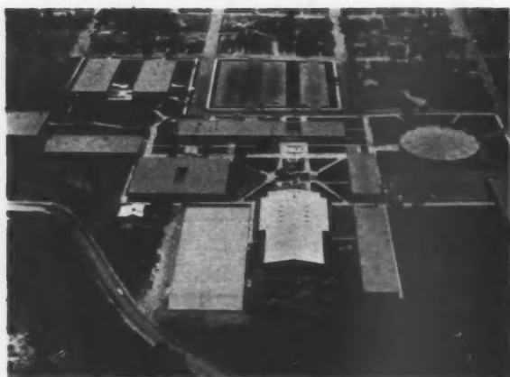
Air view of the spectacular, eleven-building campus-style high school in San Angelo, Texas
