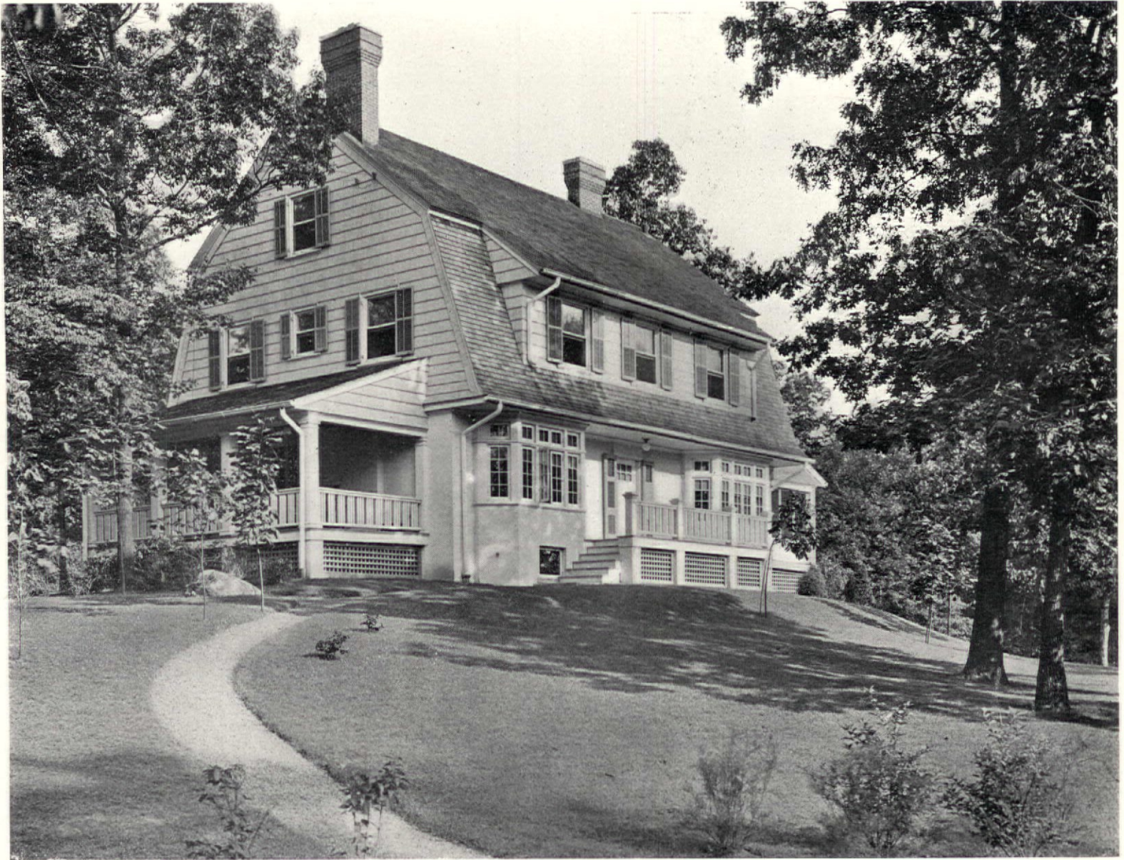
The home of Dr. Dwight E. Marvin, at Summit, New Jersey, is an unusually successful example of the gambrel roof type of house
