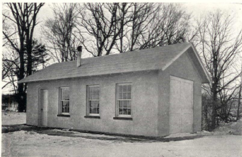
A garage and power plant can be combined, and such an equipment installed as that shown in the illustration to the right
