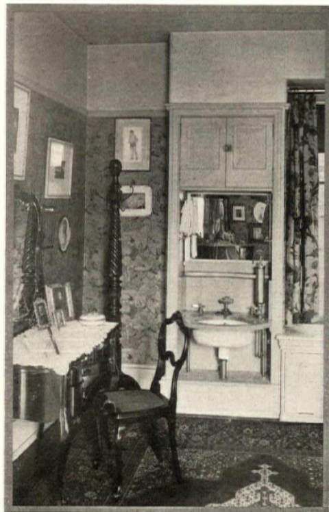
A sanitary bedroom lavatory
