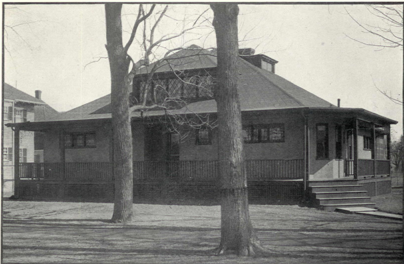
This unconventional bungalow is built of terra cotta hollow tile, covered with rough plaster, and was designed by its owners
