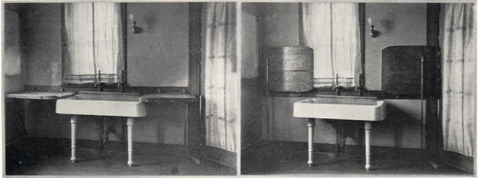
These two illustrations here shown exhibit a convenient method of arranging the drainage-boards for the well-ordered kitchen sink
