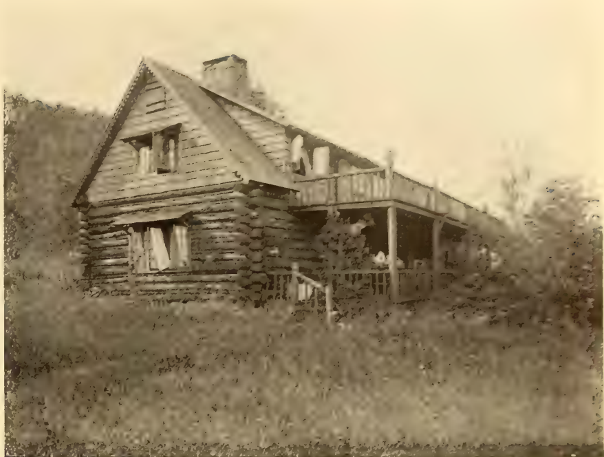
An extensive upper porch
