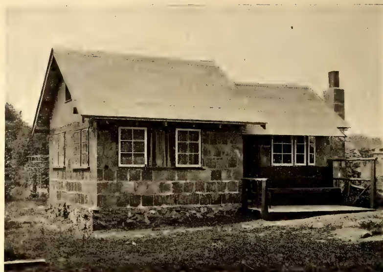
The bungalow after the extension was built
