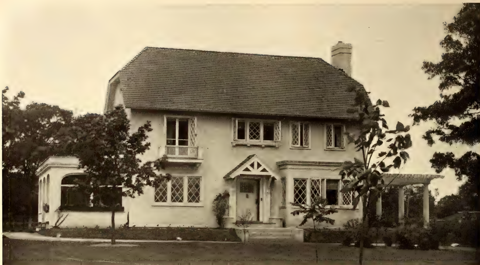
Fig. 9—The exterior walls of this house are constructed of cement stucco
