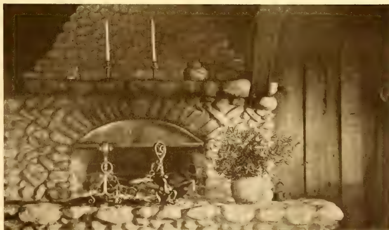
Detail of a mantel in the residence of H. B. Ainsworth, at Azusa, Cal., designed by L. B. Pemberton, architect
