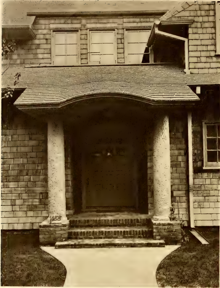
View of the front entrance which shows the steps formed of brickwork and the pillars of concrete. The roof is supported by the pillars which shelter the front door, and above the latter are three small windows which provide light to the hall and the stairway
