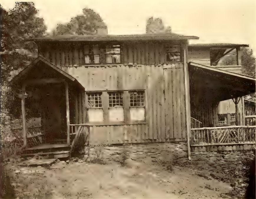
Perpendicular slabs are used
