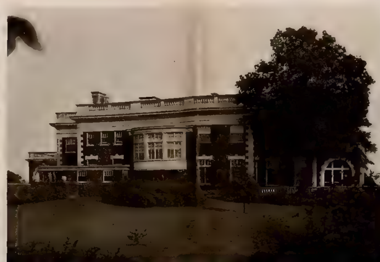
The rear of the house
