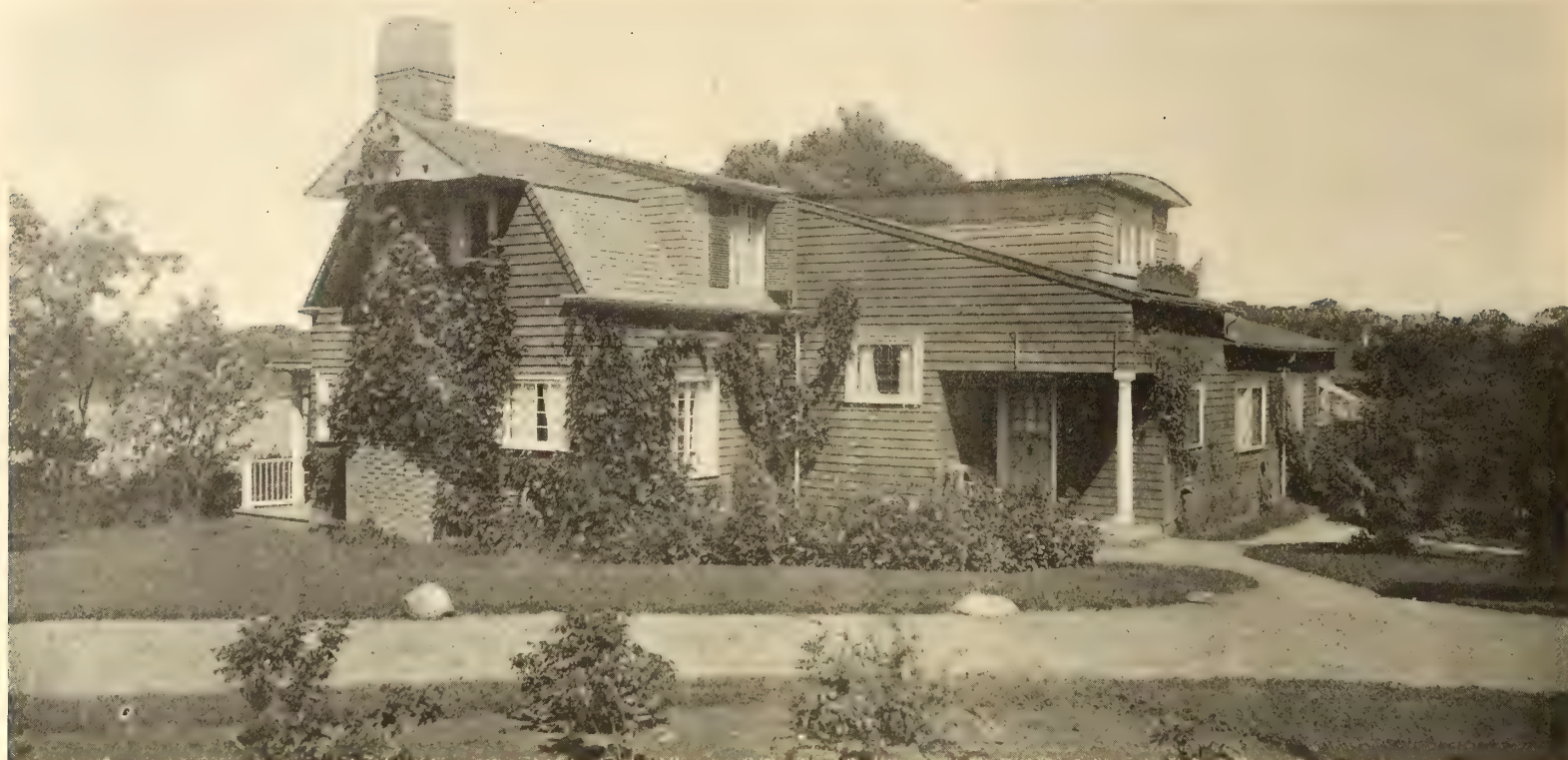
The old Bunk House made into a full-grown cottage
