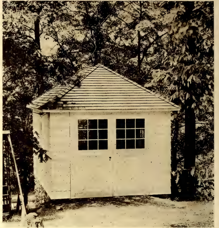
The country dweller who does not wish to go to great expense, may well erect a little garage of this sort
