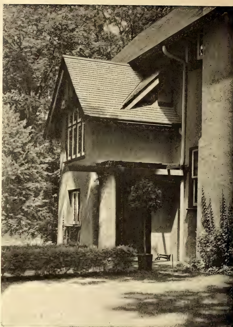
Main entrance of the building
