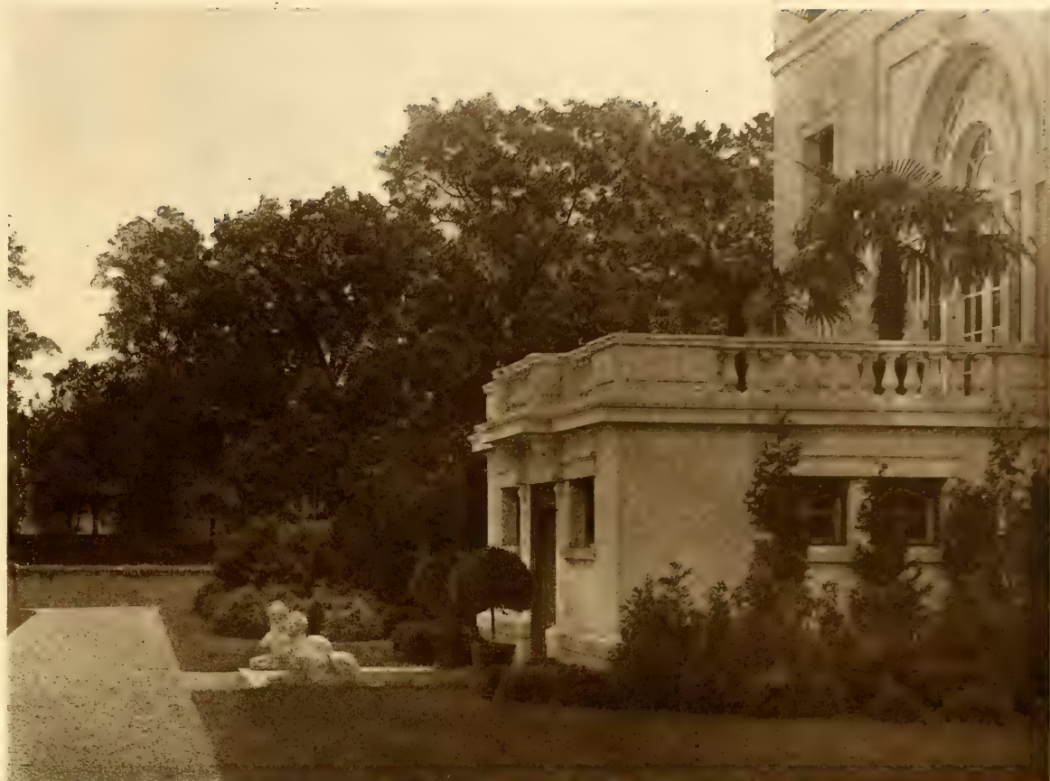
The entrance to the north front
