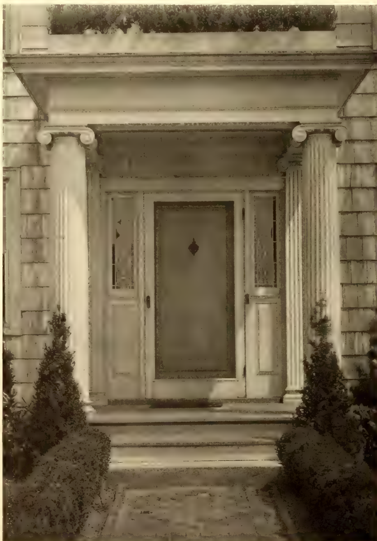
Fig. 1—The classic porch at the front of the house
