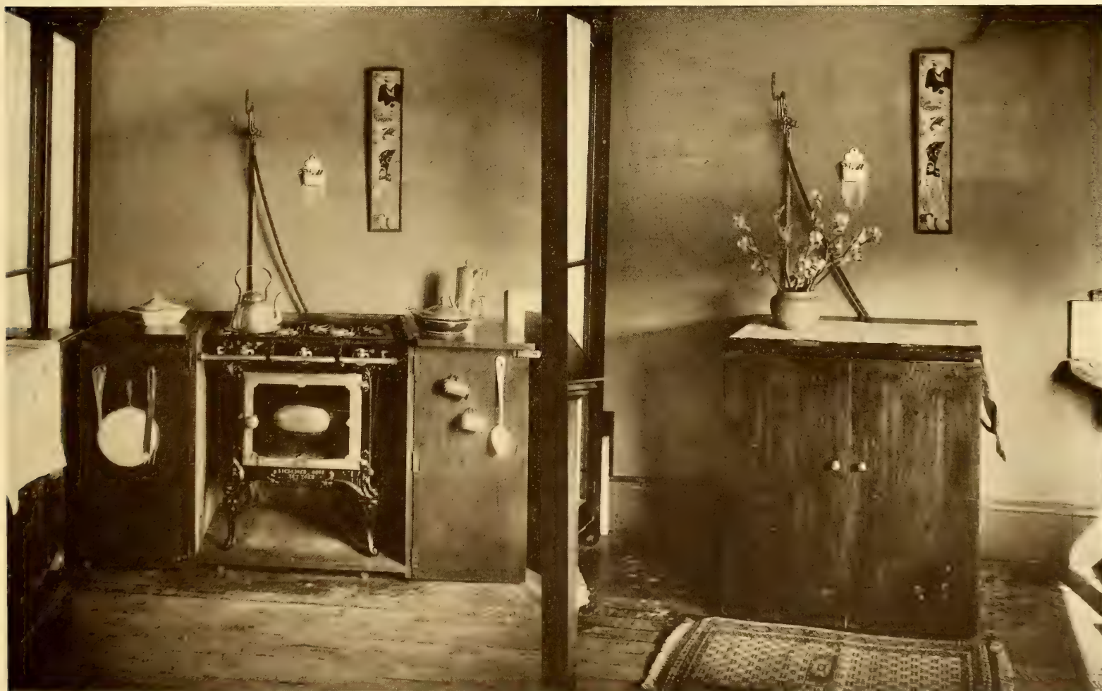
This shows kitchenette cupboard, open and ready for use
