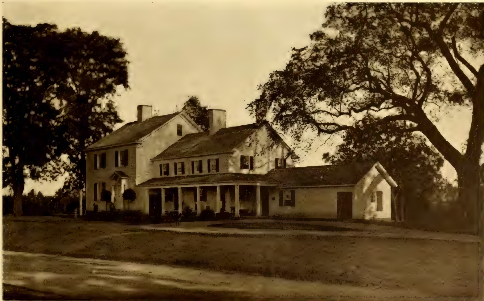
The remodeled house of Dr. Fahnestock, and the newly graded lawn with all the striking difference from the old form, required very slight changes
