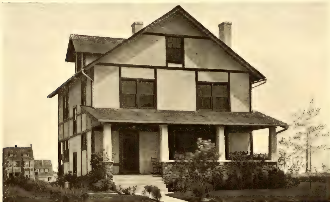
Fig. 26—A house of simple construction
