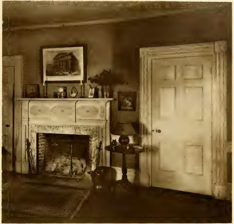
Old woodwork in the living-room of Mr. Olcott's house
