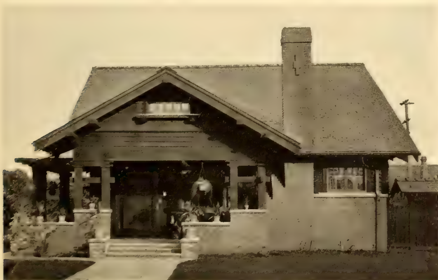
Fig. 15—The porches are connected by a terraced wall
