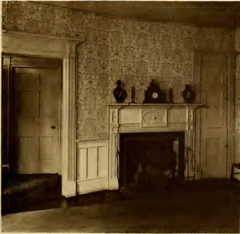
A corner of the dining-room of Mr. Olcott's house
