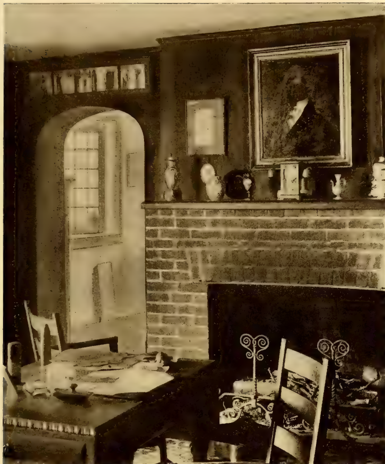
A corner of the library, showing the newly constructed fireplace
