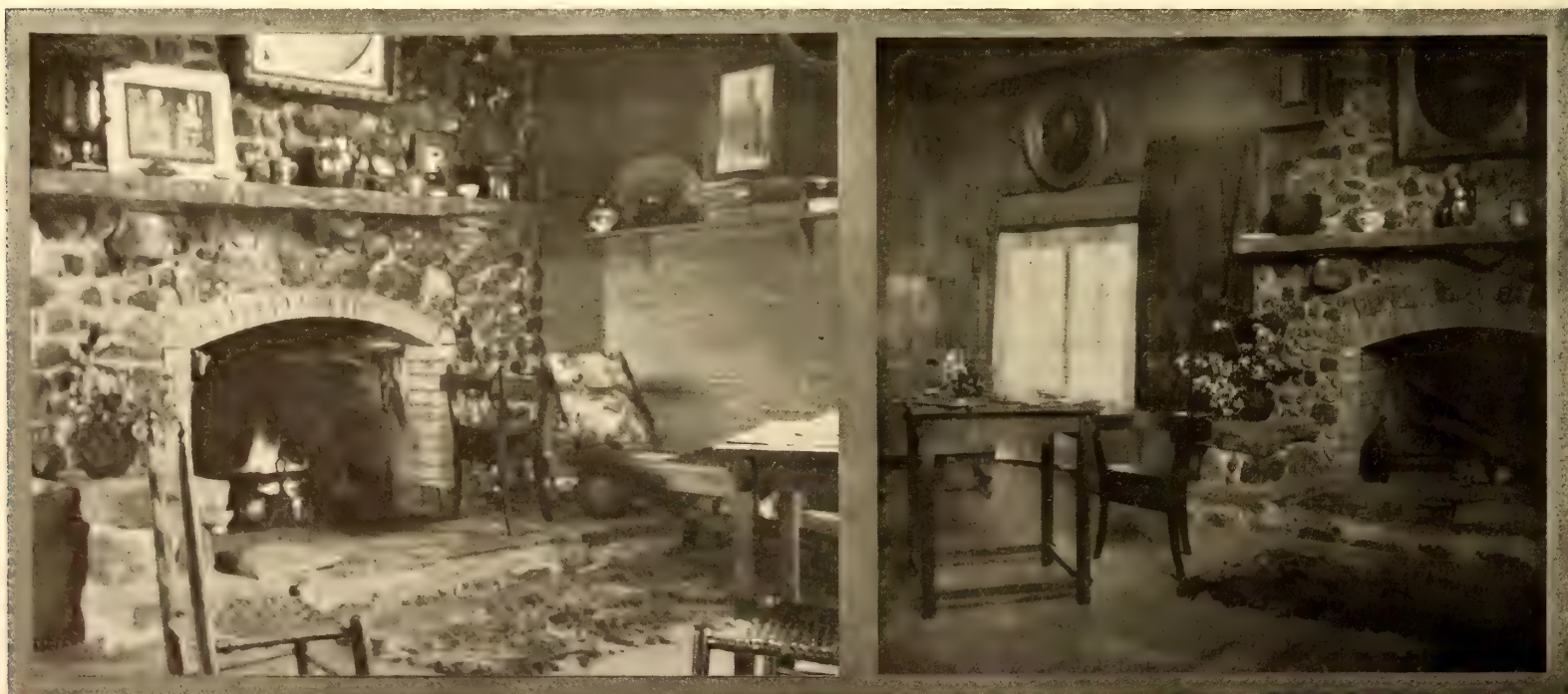
These two views of the studio-room chimney corner at "Laurel Lodge" show the possibilities of rough cobbles used for interior building purposes
