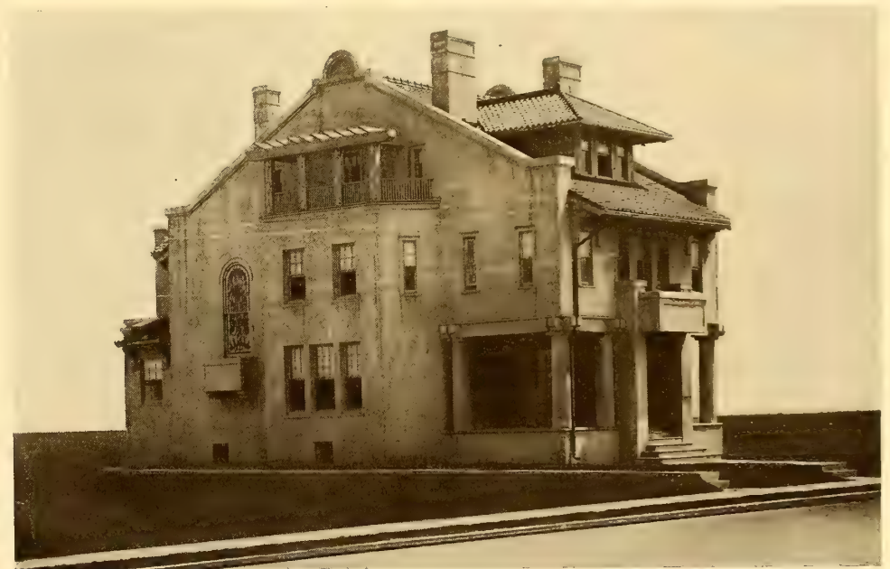
Fig. 25—Cement is used with a restraining effect
