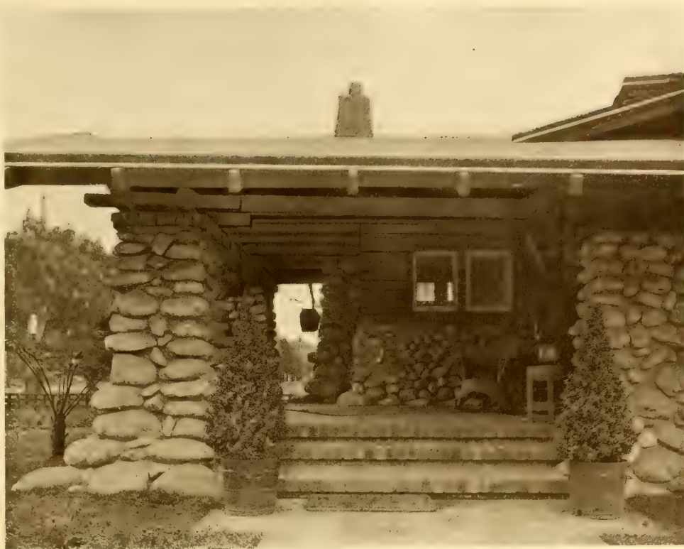
The front walk, which enters Mr. Parsons' bungalow at the side. The walk is of brick, as well as the steps leading to the porch
