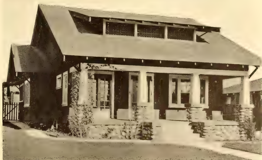
Fig. 16—Field stone and shingles are the materials used. Cost, $1,900
