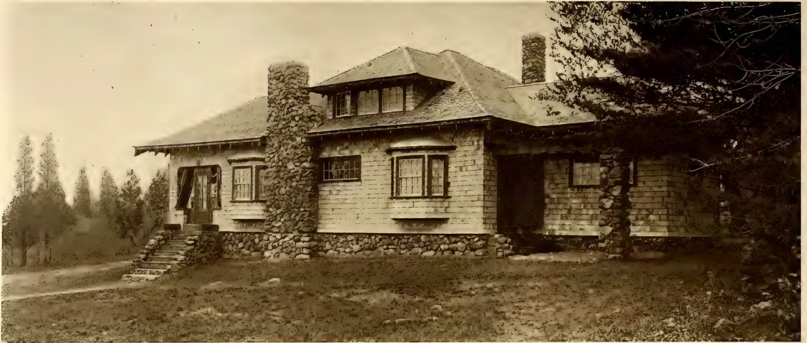
Field stone and shingles are the materials used for the exterior walls
