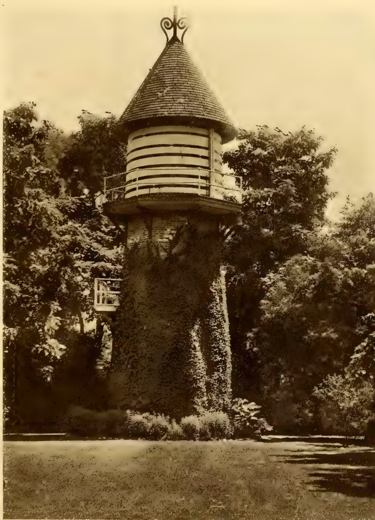
Fig. 1—A brick tower and wooden tank
