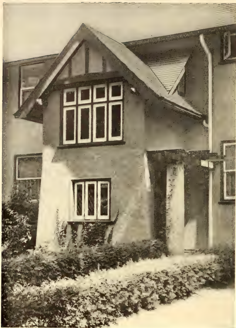
Exterior wall of the staircase
