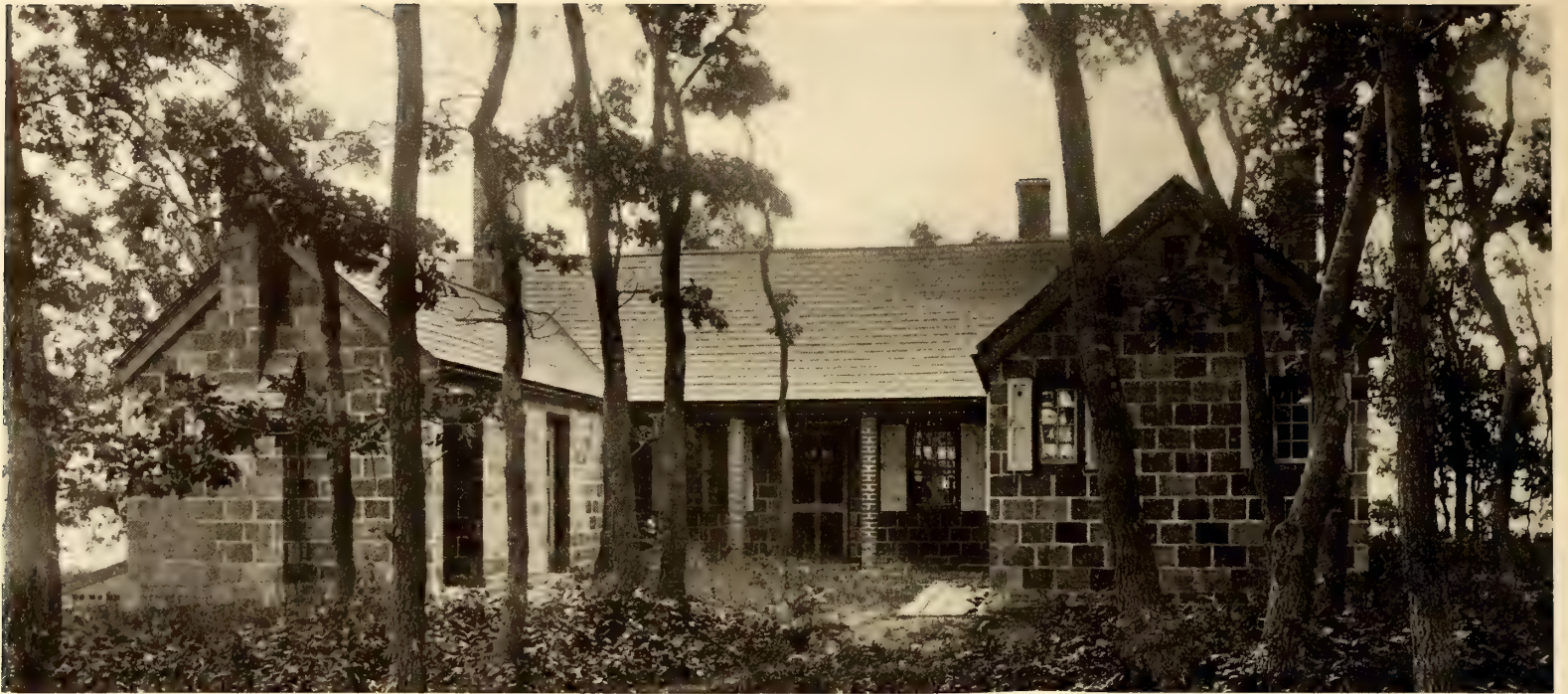
The rear of the house showing the court
