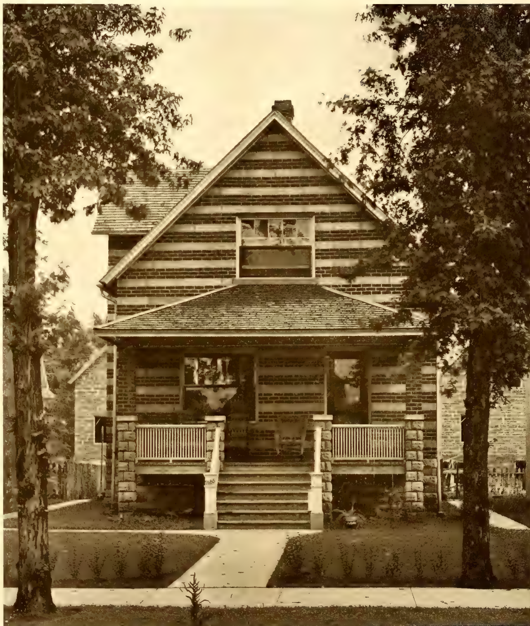
A home of stone and brick
