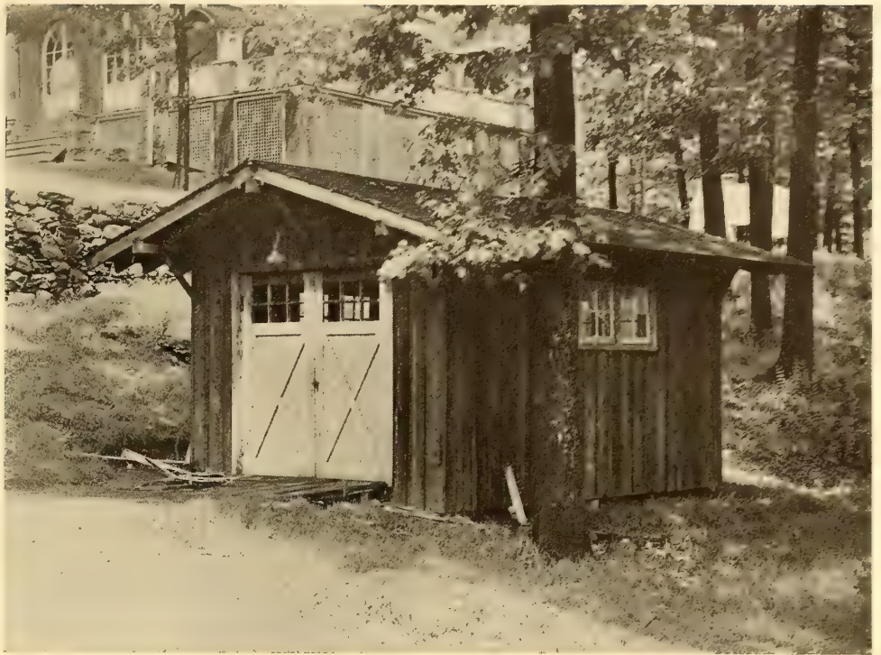
A garage built of log slabs on a wooden framework
