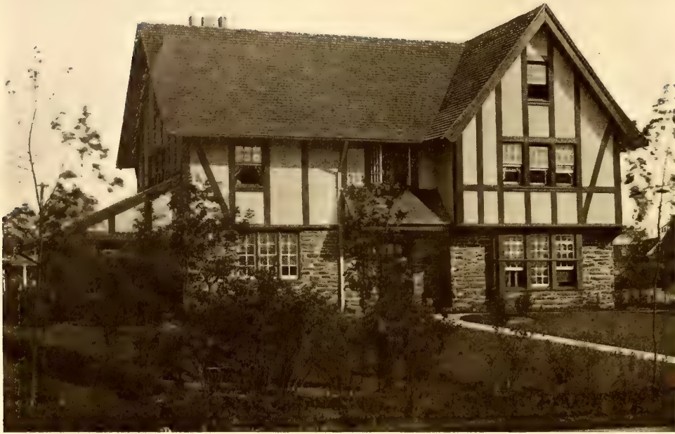
A stone and half-timber house
