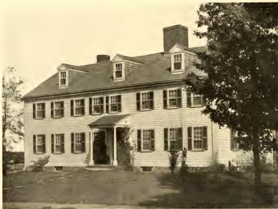
Mr. Walter Scott Hopkins' house, at Reading, Mass., after the alterations
