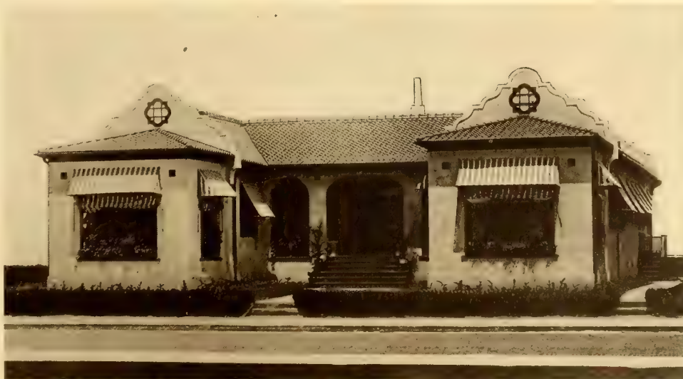
Fig. 2—A home of bungalow construction
