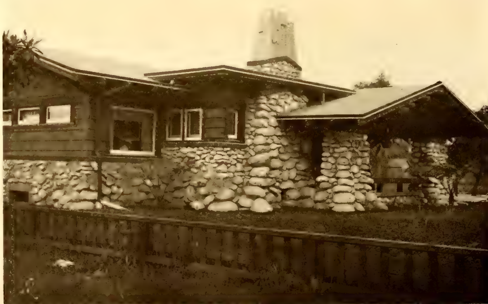
In Mr. Parsons' bungalow, cobblestones, brick and plaster are employed, with the walls above shingled. Each second course of shingles is exposed, with a one-half inch strip beneath to produce a more rustic effect. Note the heavy timber of the head casing, which runs around the building just above the windows, and which accentuates the low, long bungalow lines
