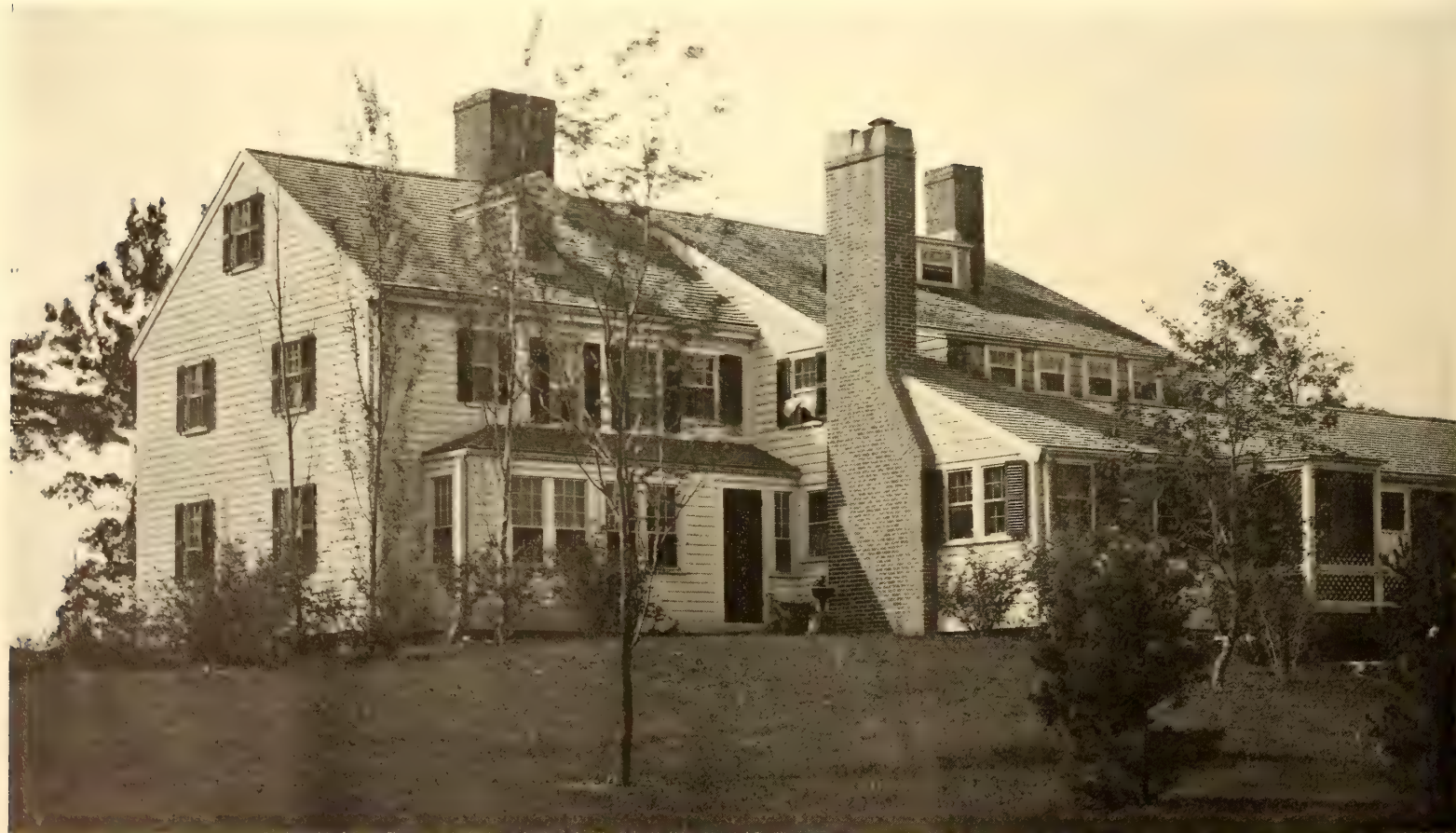
Garden side of Mr. Walter Scott Hopkins' house, showing the long, sweeping roof reaching almost to the ground, as in the old house
