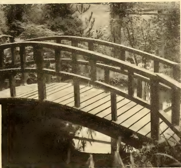
A plain type of wooden bridge
