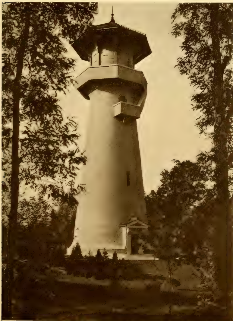
Fig. 8—A stucco tower with the tank surrounded by a balcony
