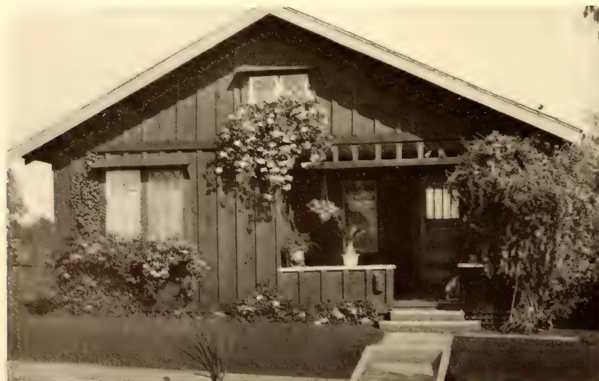
Fig. 9—A bungalow of simple design and construction. Cost, $800
