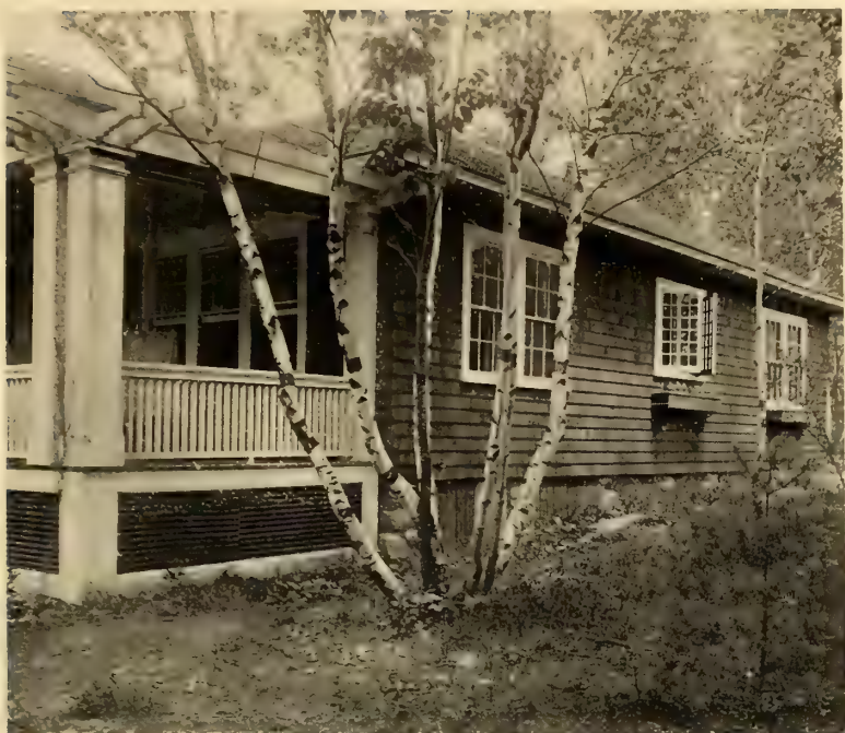
Side view of the Archer bungalow, showing casement windows
