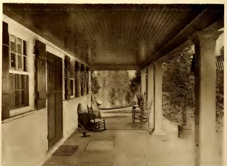
The interior of the porch
