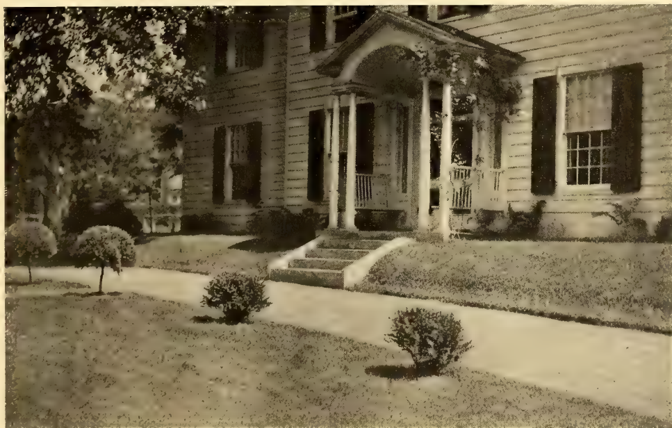
House of Mr. Howard McWilliams of Plainfield, New Jersey, along old-time lines
