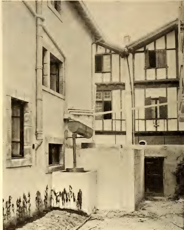
Showing the pipes during the rain
