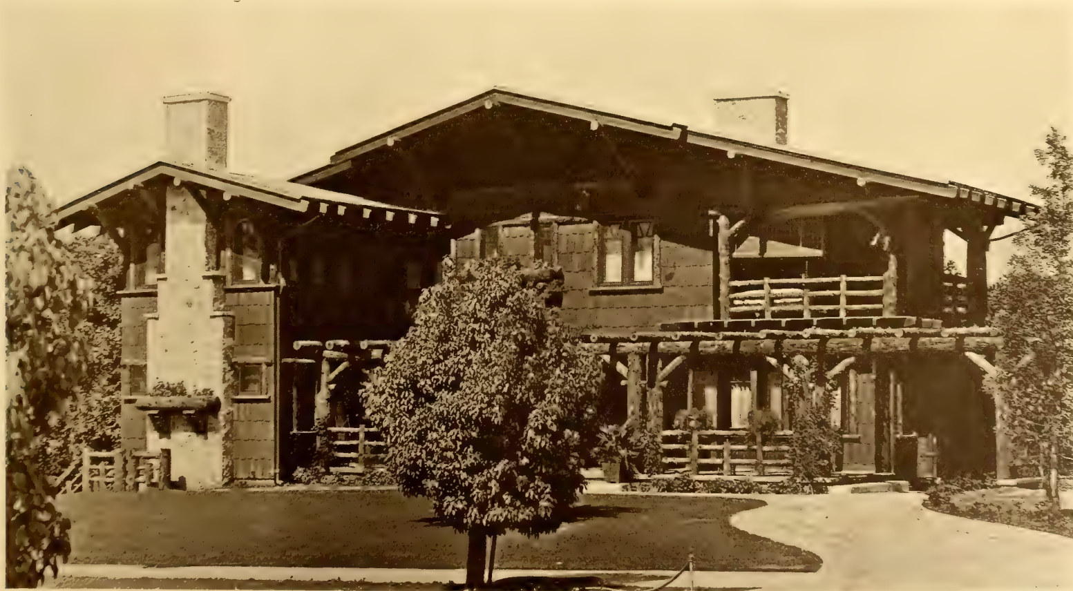
The characteristics of the Swiss chalet are revealed in this house
