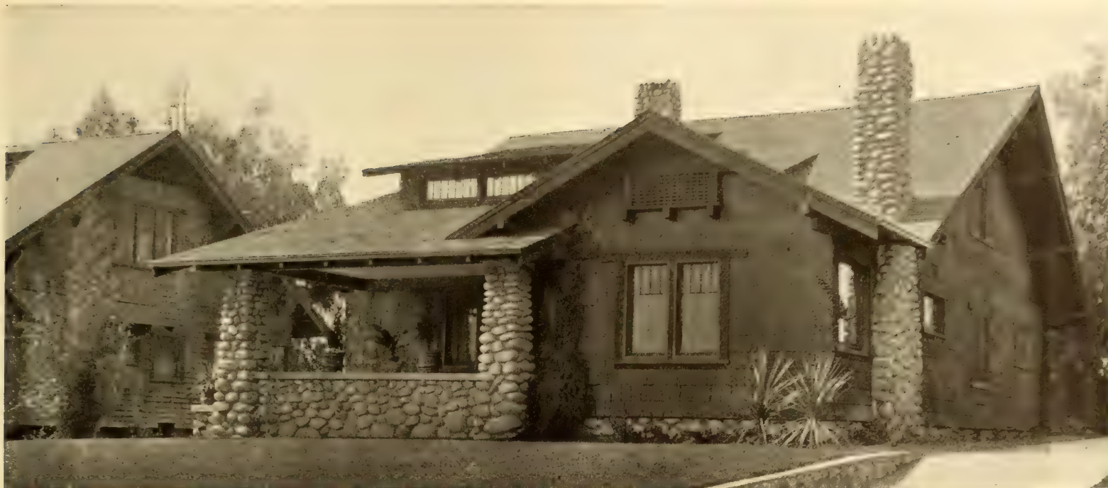
Fig. 1—Cobblestones and brown-stained shingles are used for the exterior of this bungalow
