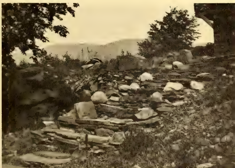
The kitchen approach to "Laurel Lodge" is partly up these steps, that have been made of stones hewn from the little quarry at their side
