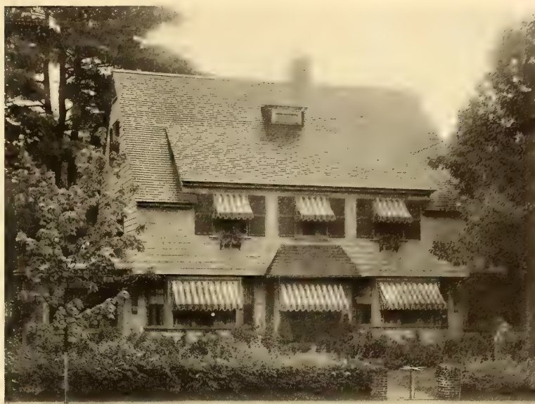
A shingled house of good design
