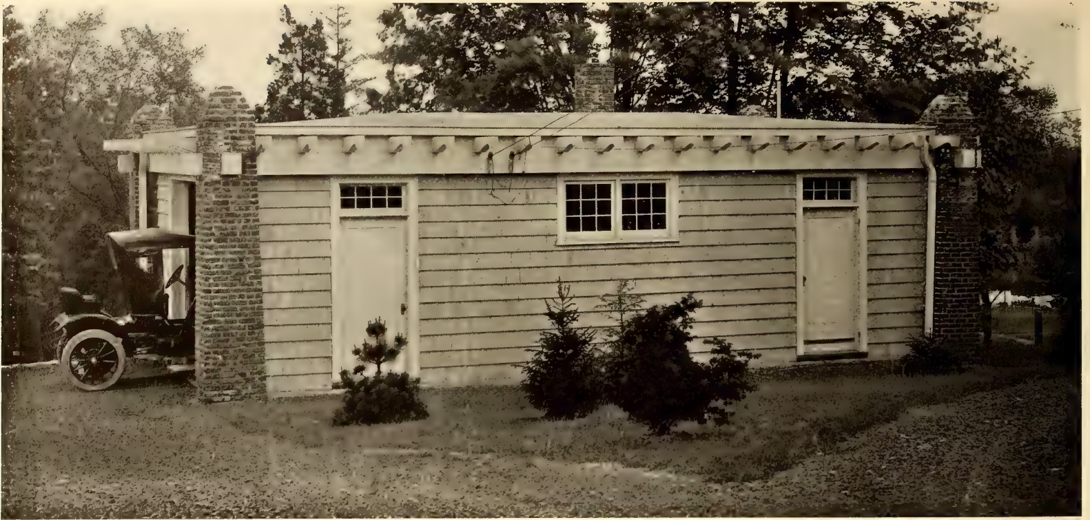
A garage built of shingles. The flat roof prevents obstruction of view from the house
