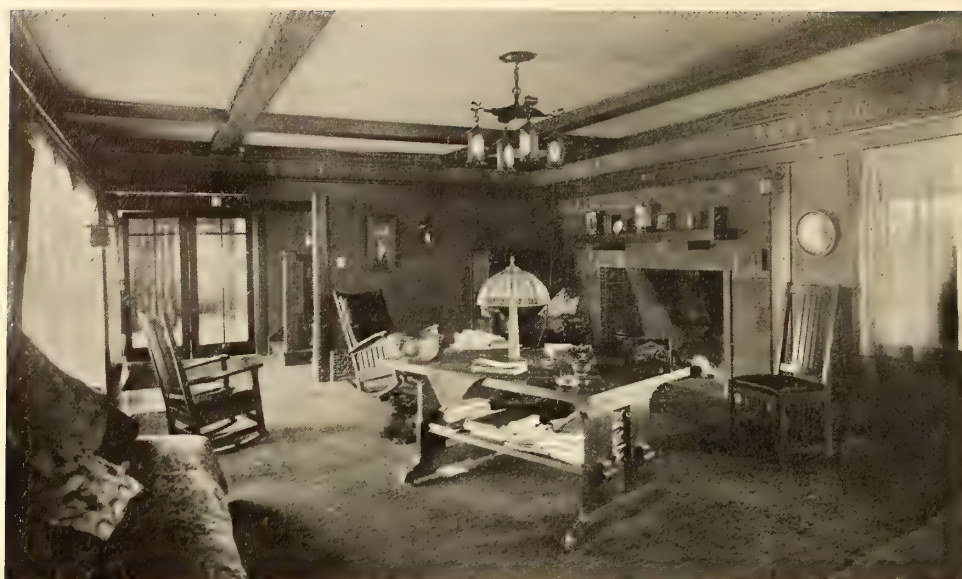
Fig. 1—Dining-room with tile and brick semi-ingenook fireplace. The head casing runs around the room, forming a frieze panel
