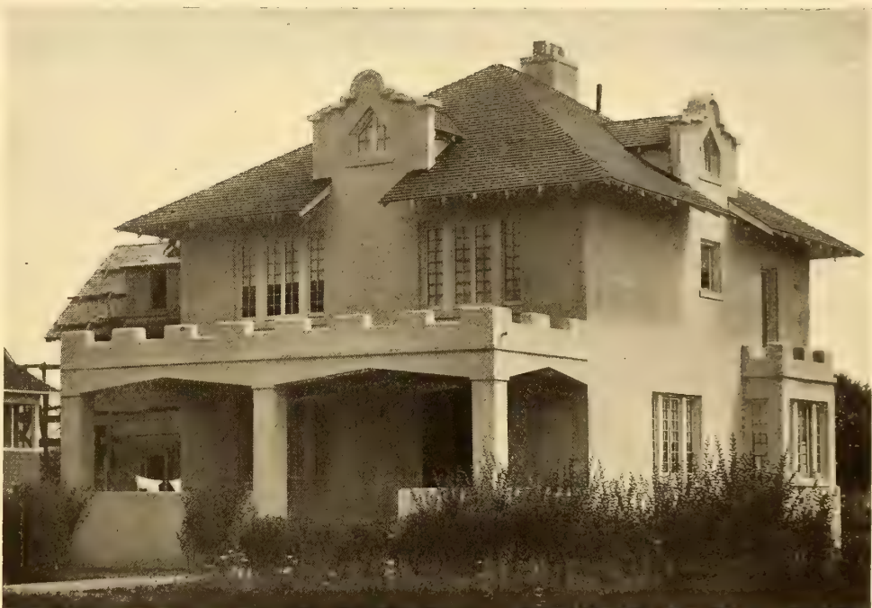
Fig. 15—A house built of hollow tile
