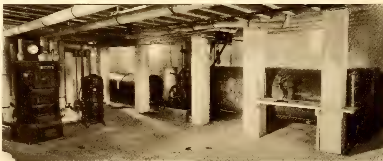
The larger tank is supplied from the well containing hard water; the smaller one from a cistern containing soft water
