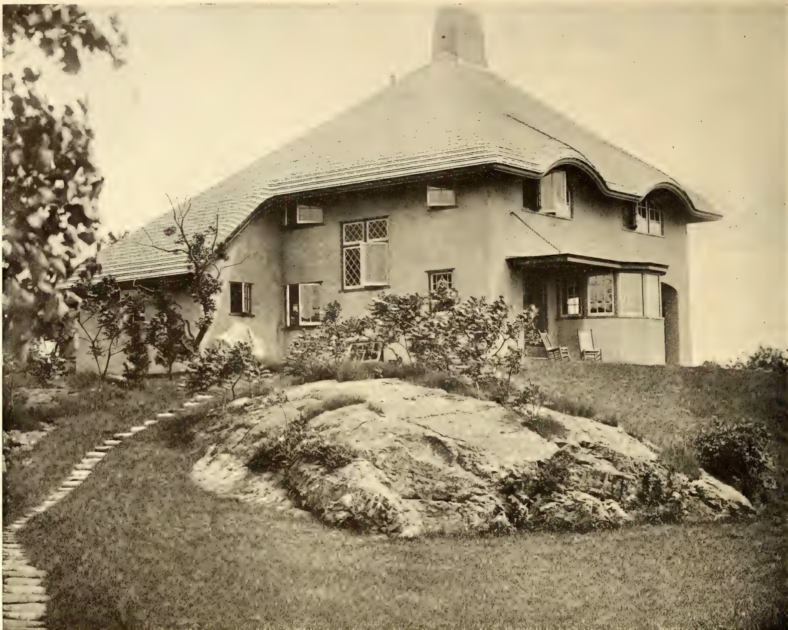
This picturesque cottage is one of the most successful examples in American small house architecture, both in its design and careful planning
