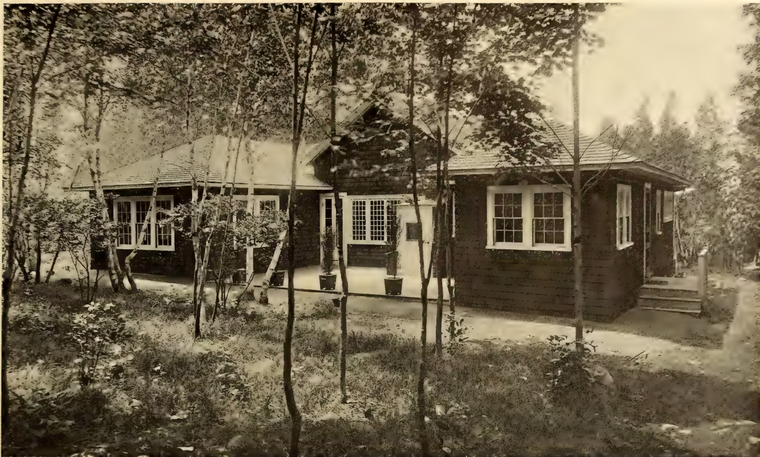
Front view of the Archer bungalow
