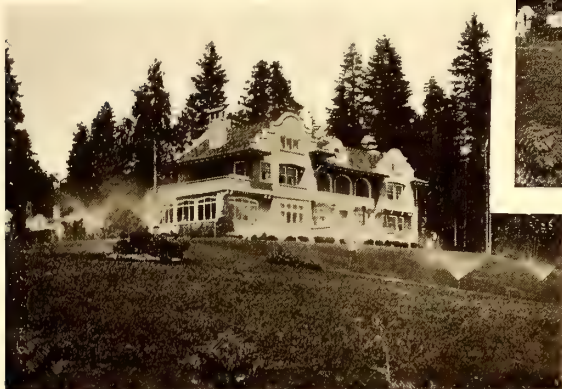
Spraying the lawn by pneumatic pressure
