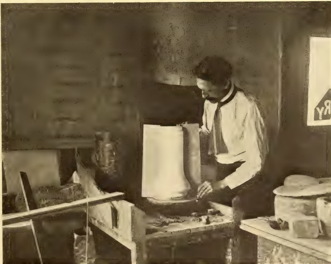
Preparing to build up the two halves of the mold about the model.
