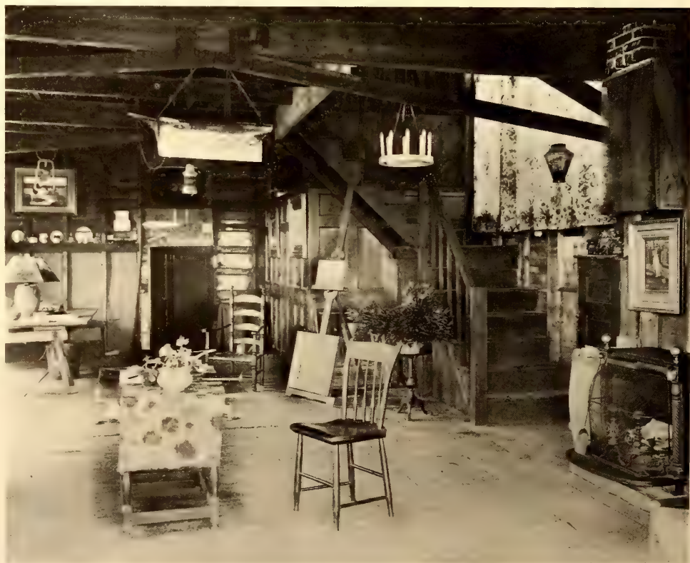
The interior of the boathouse as it is
