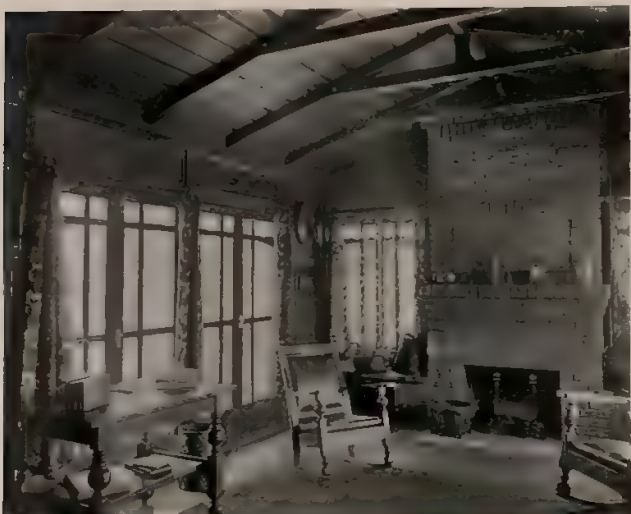
Fig. 2—Mahogany red and brown wood stain in a bungalow in which all the construction (roof, walls, etc.) is exposed
