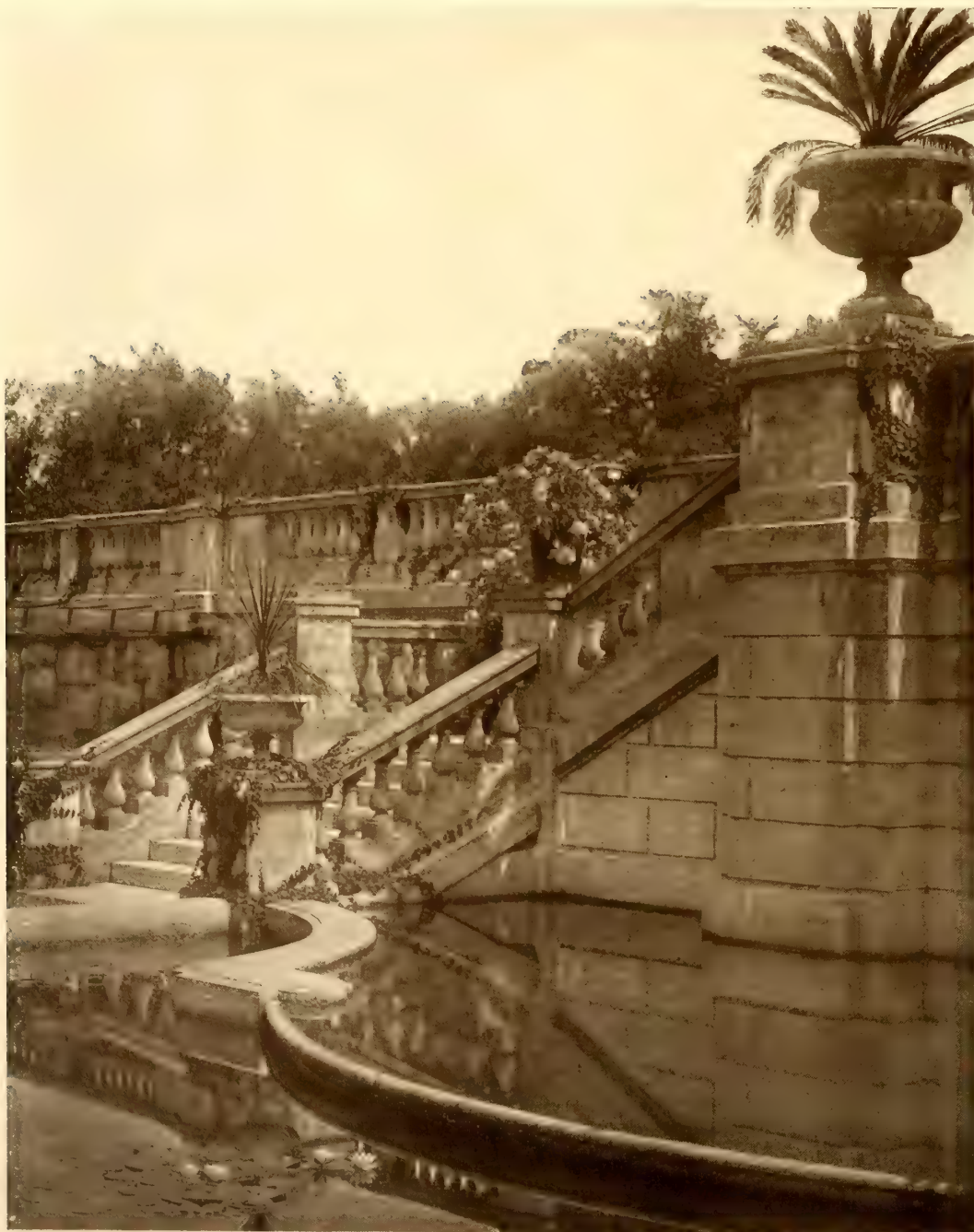
The balustrade and steps to the water garden
