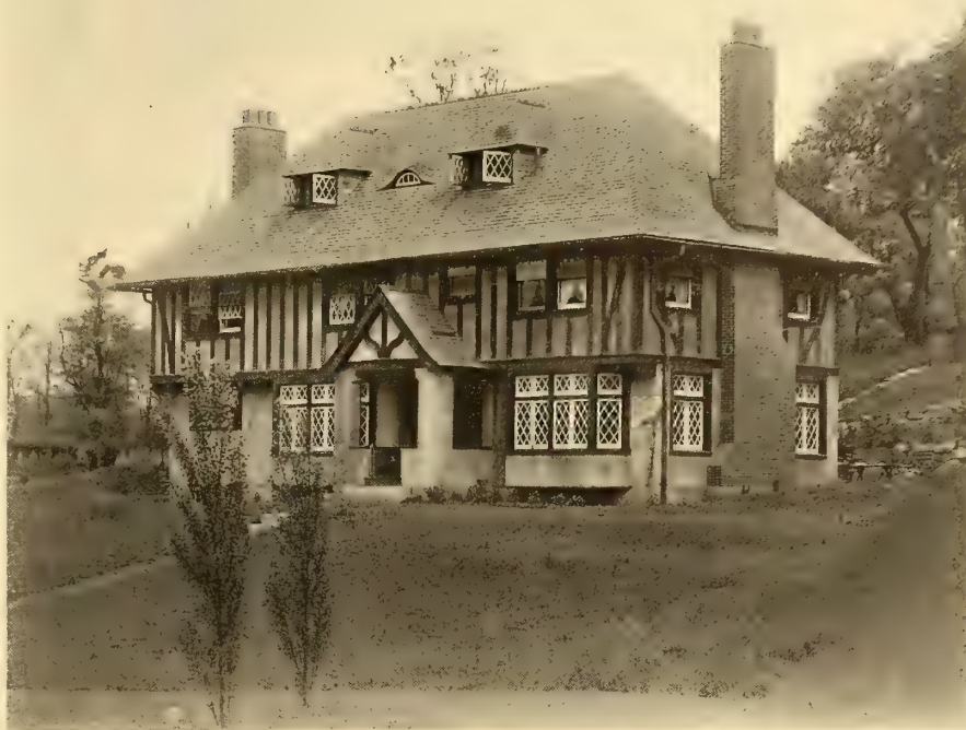
Fig. 11—A house of stucco and half-timber wood
