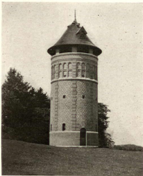
Fig. 2—A brick tower with the tank hidden by the wall
