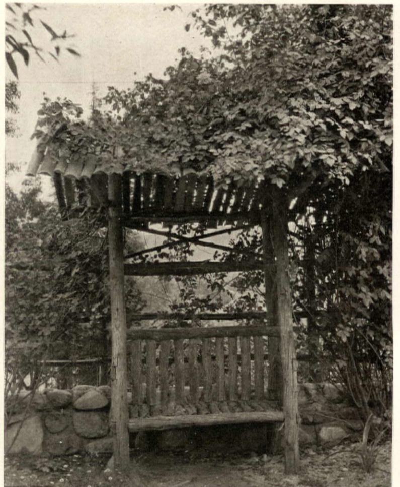
Rustic garden seat of eucalyptus. Roof thatched with stems of palm leaves
