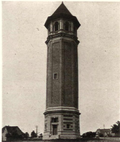
Fig. 5—Brick and stone tower with tank in the enclosure at top
