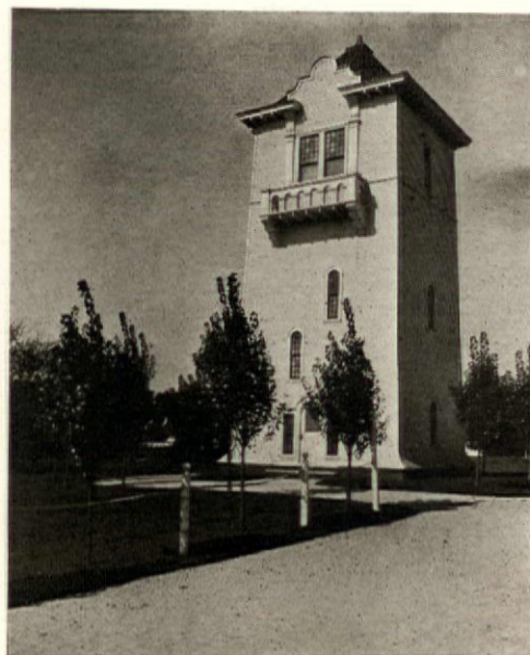
Fig. 3—A wooden tower with the tank hidden by the wall
