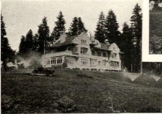
Spraying the lawn by pneumatic pressure
