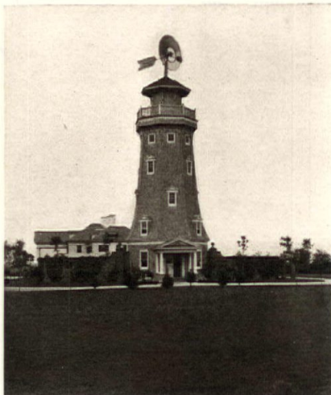
Fig. 6—The tank and windmill is built on top of the tower
