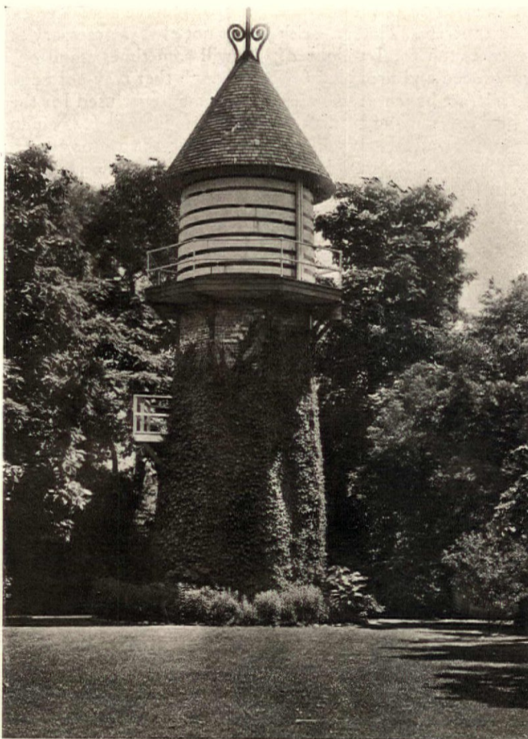
Fig. 1—A brick tower and wooden tank
