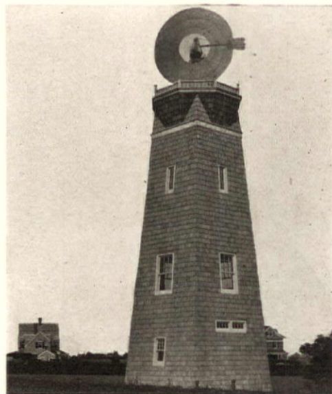
Fig. 7—A wooden tower with windmill at top and tank enclosed underneath
