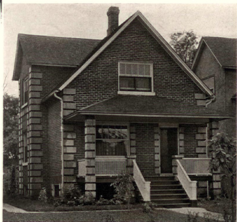
A brick and cement block house. Cost $3,300
