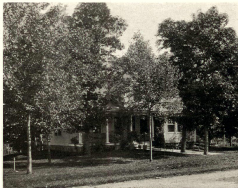
Two pneumatic tanks are installed in the basement of this house
