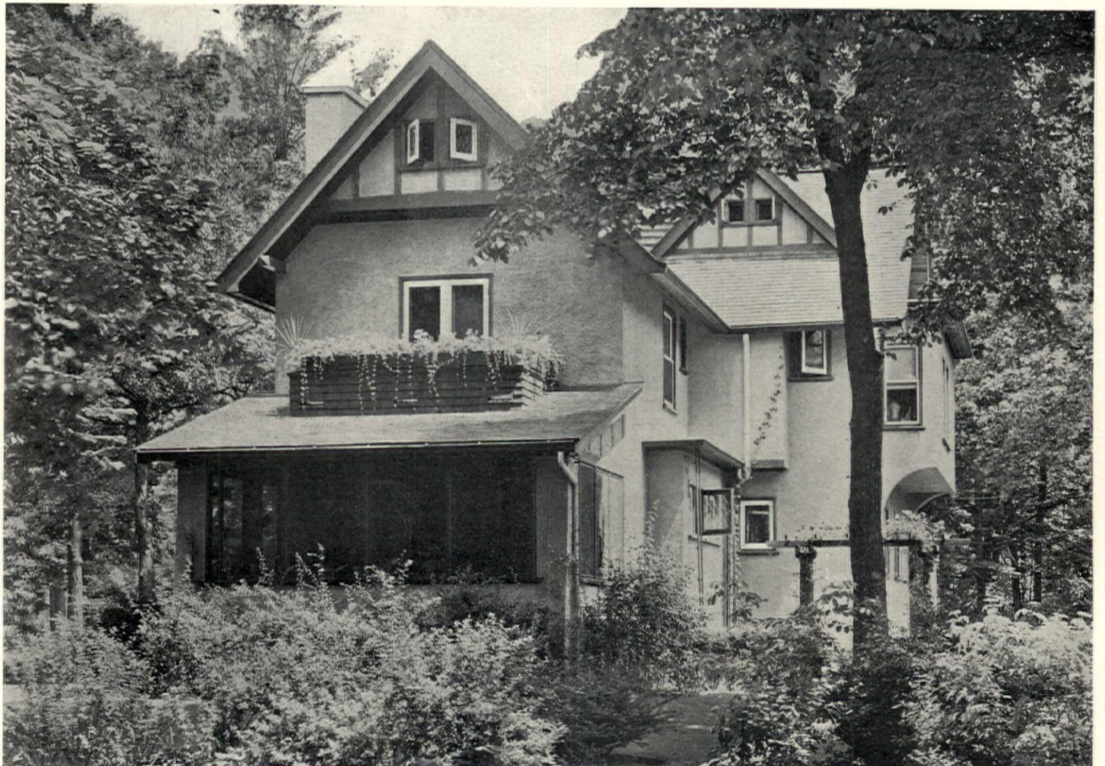
The side and rear of the house
