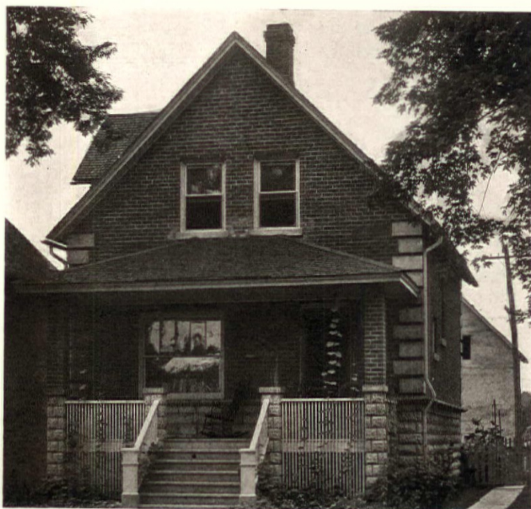
A brick and cement block house. Cost $3,300
