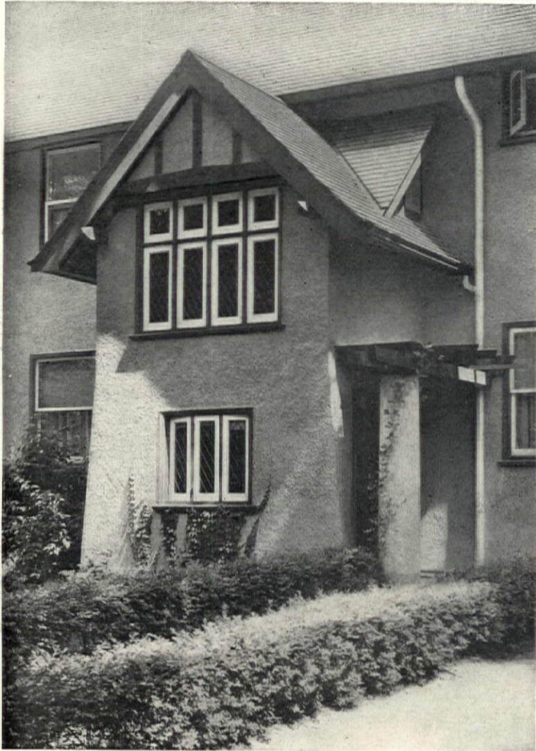
Exterior wall of the staircase
