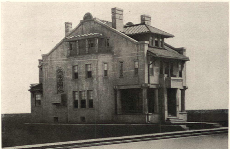
Fig. 25—Cement is used with a restraining effect
