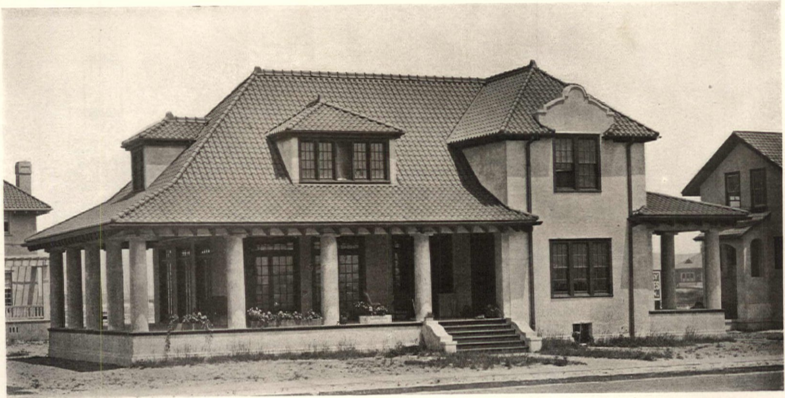
Fig. 7—The red tile roof and the stucco walls mingle finely together
