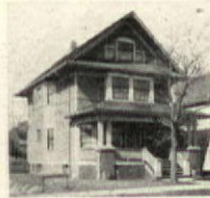
A No. A-241 IDEAL Boiler and 461 ft. of 38-in. AMERICAN Radiators, costing owner $215, were used to heat this cottage.
