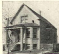
A No. 2118 IDEAL Boiler and 270 ft. of 38-in. AMERICAN Radiators, costing owner $135, were used to heat this cottage.
