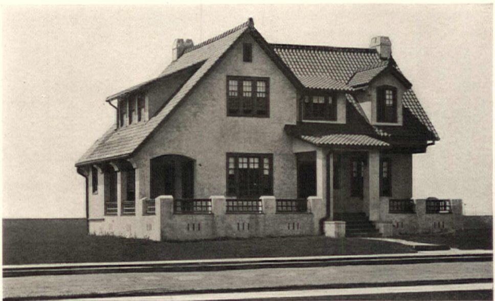
Fig. 22—A design of a true concrete house
