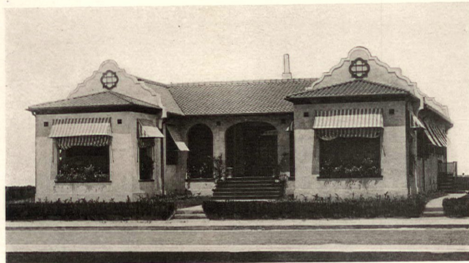
Fig. 2—A home of bungalow construction
