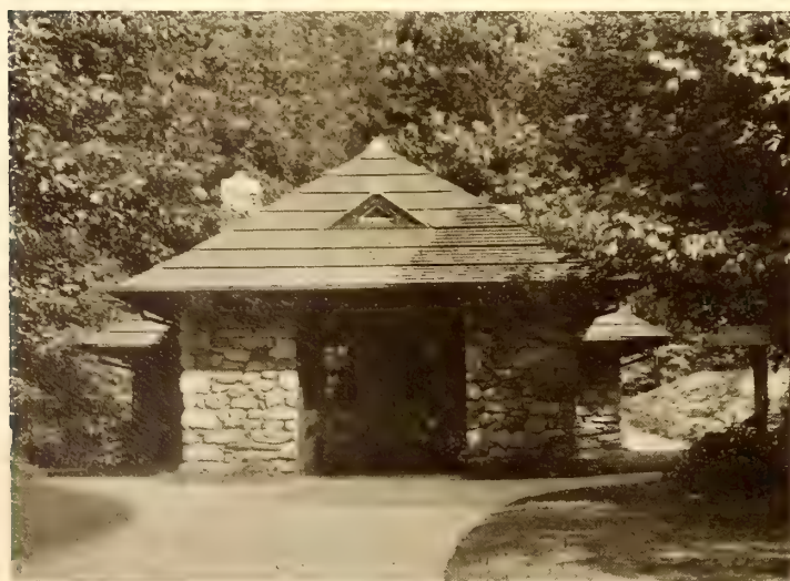
The Pump House for the Water Supply
