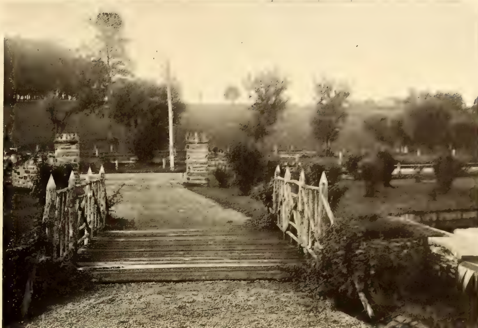
Bridge Roadway with Rustic Railing
