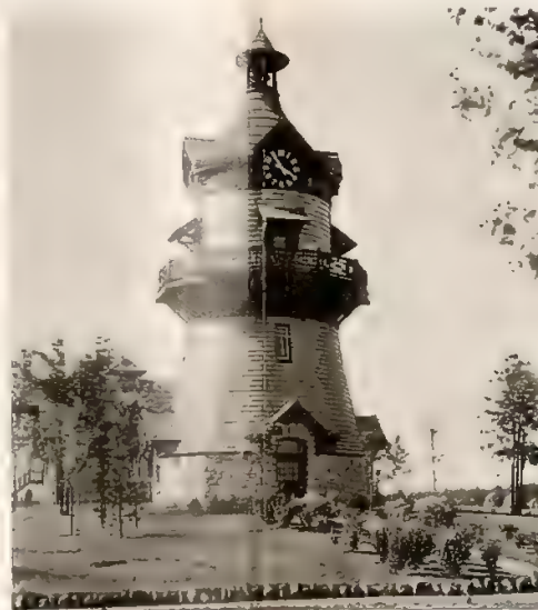
Clock and Water Tower
