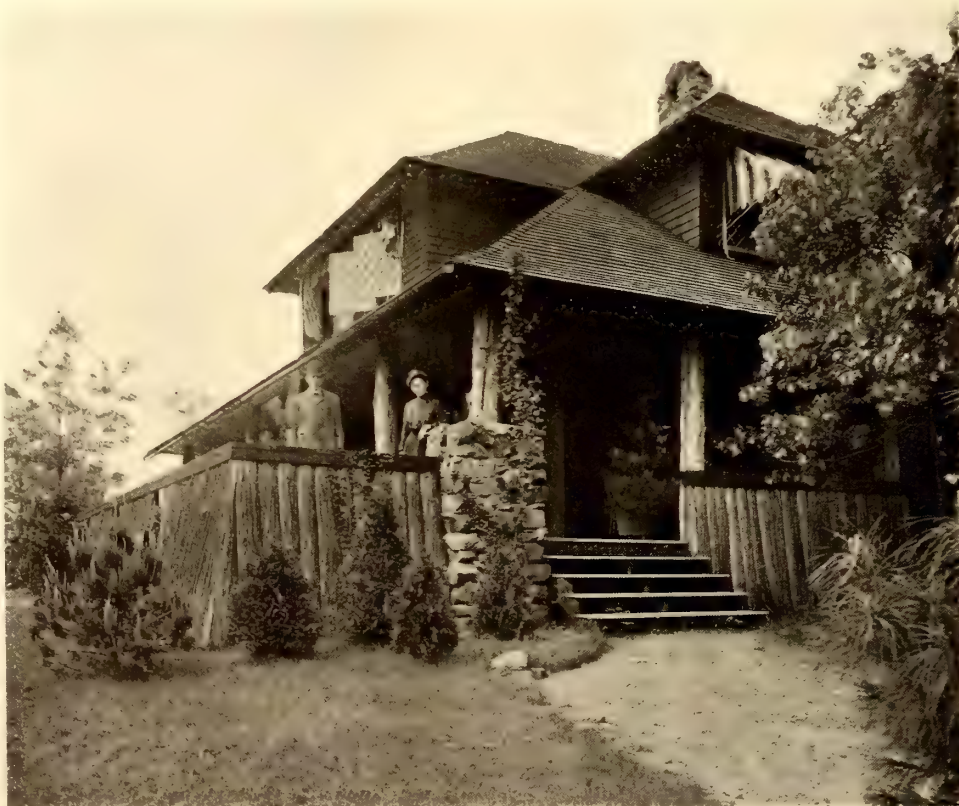
The Four Corners of the House Rest on Fieldstone Piers
