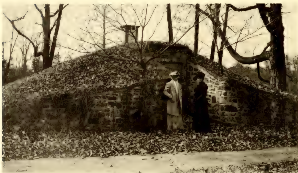
Dome-shaped Spring-House at Andalusia
