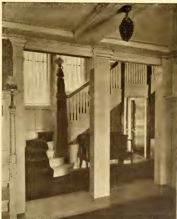
The Staircase Hall
