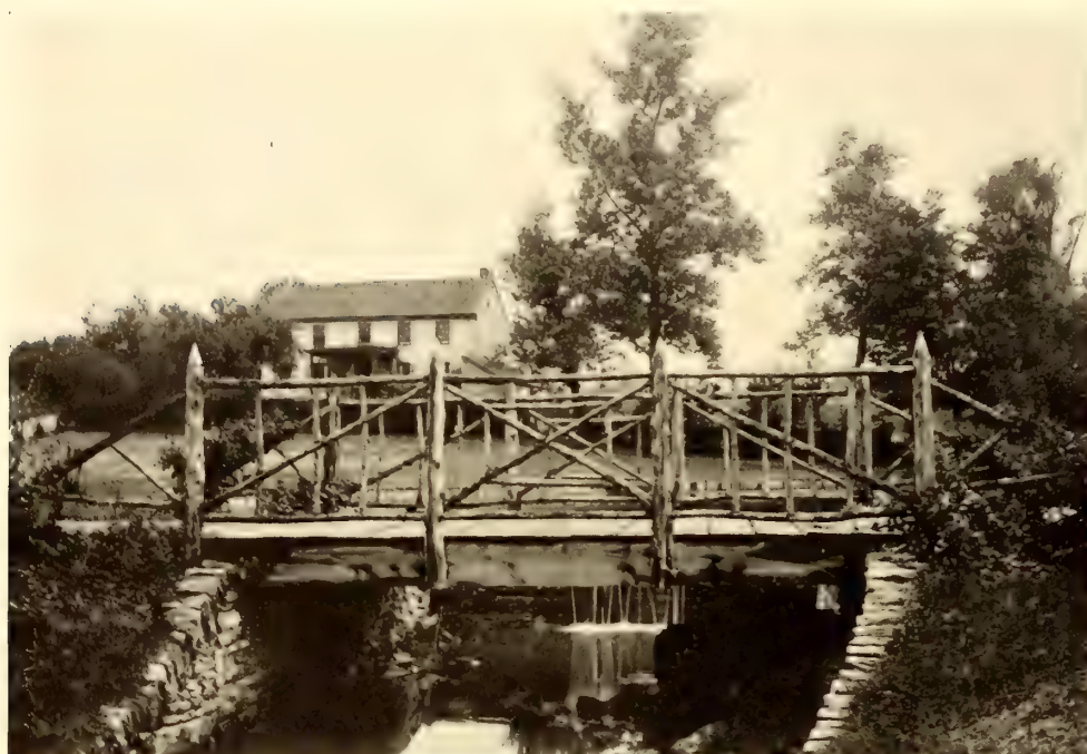
A Rustic Bridge of Simple Design
