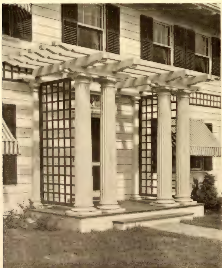
The Pergola-like Porch of the Entrance Door
