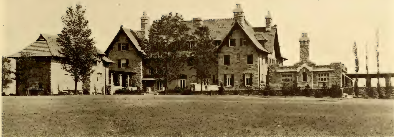
The Casino, Manor House and Dining-room
