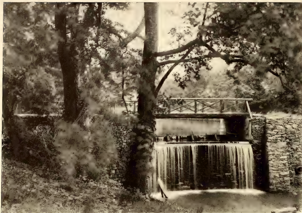
Bridge Above a Dam
