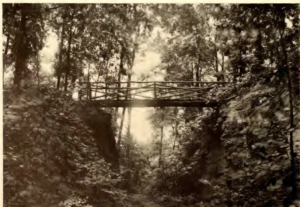
A High Bridge Across a Stream
