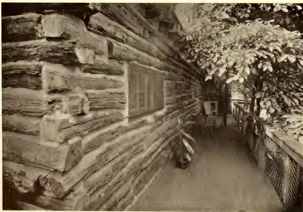
The Porch Above the Creek
