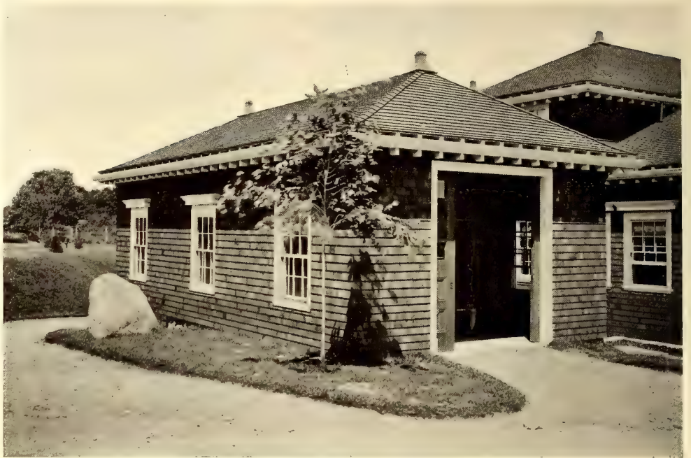
Garage Design in Harmony with the House
