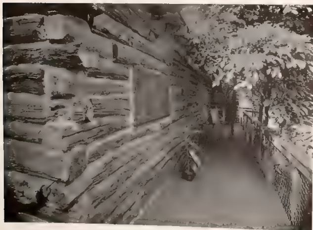
The Porch Above the Creek
