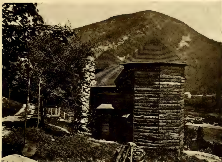
A Form of Slab Building Which Is Common but Which Should Be Avoided
