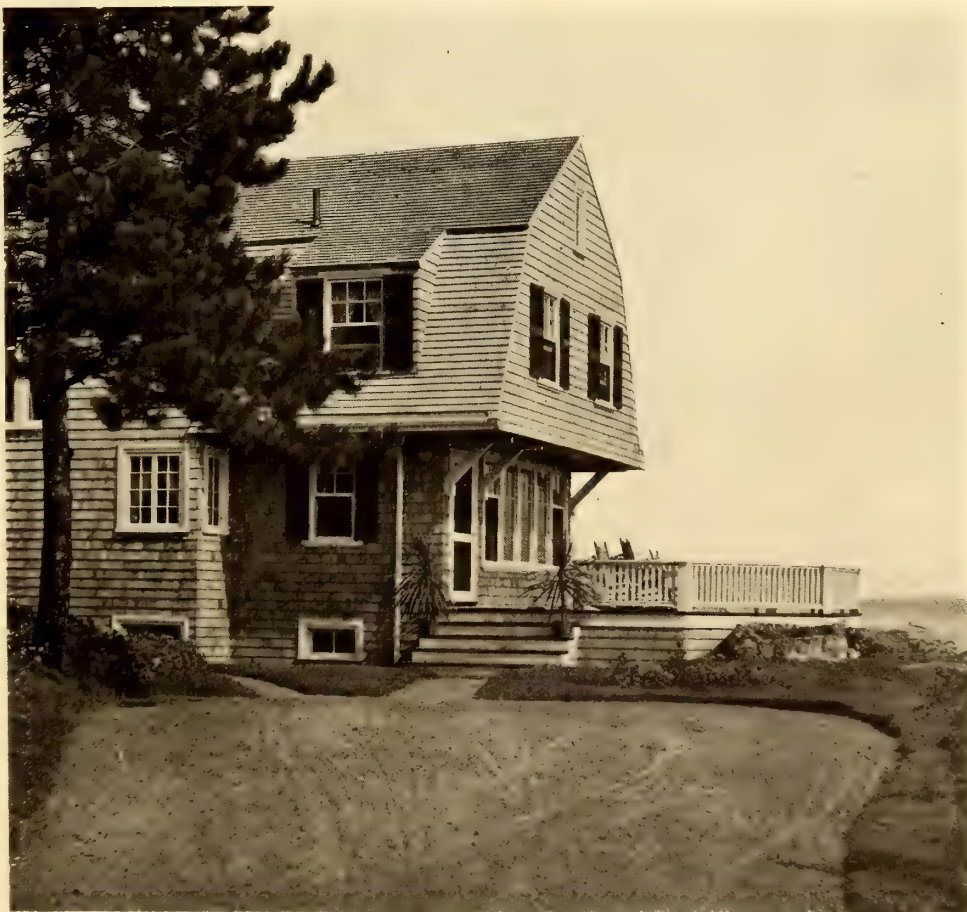
Gable End and Terrace
