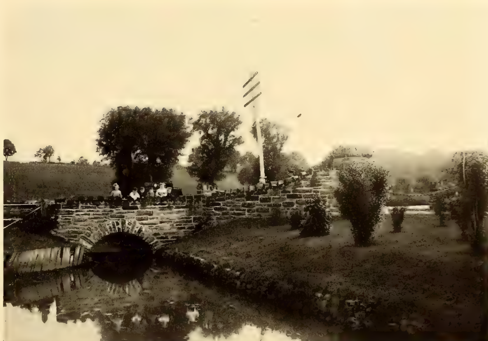
Entrance Bridge Across a Public Highway
