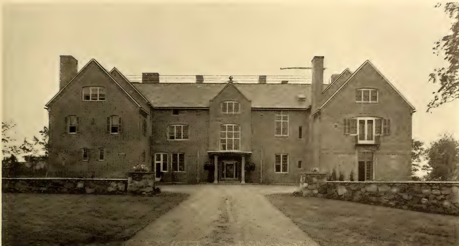
The House Is Built of Harvard Brick, with Bands and Ornaments of Brightly Colored Mercer Tiles
