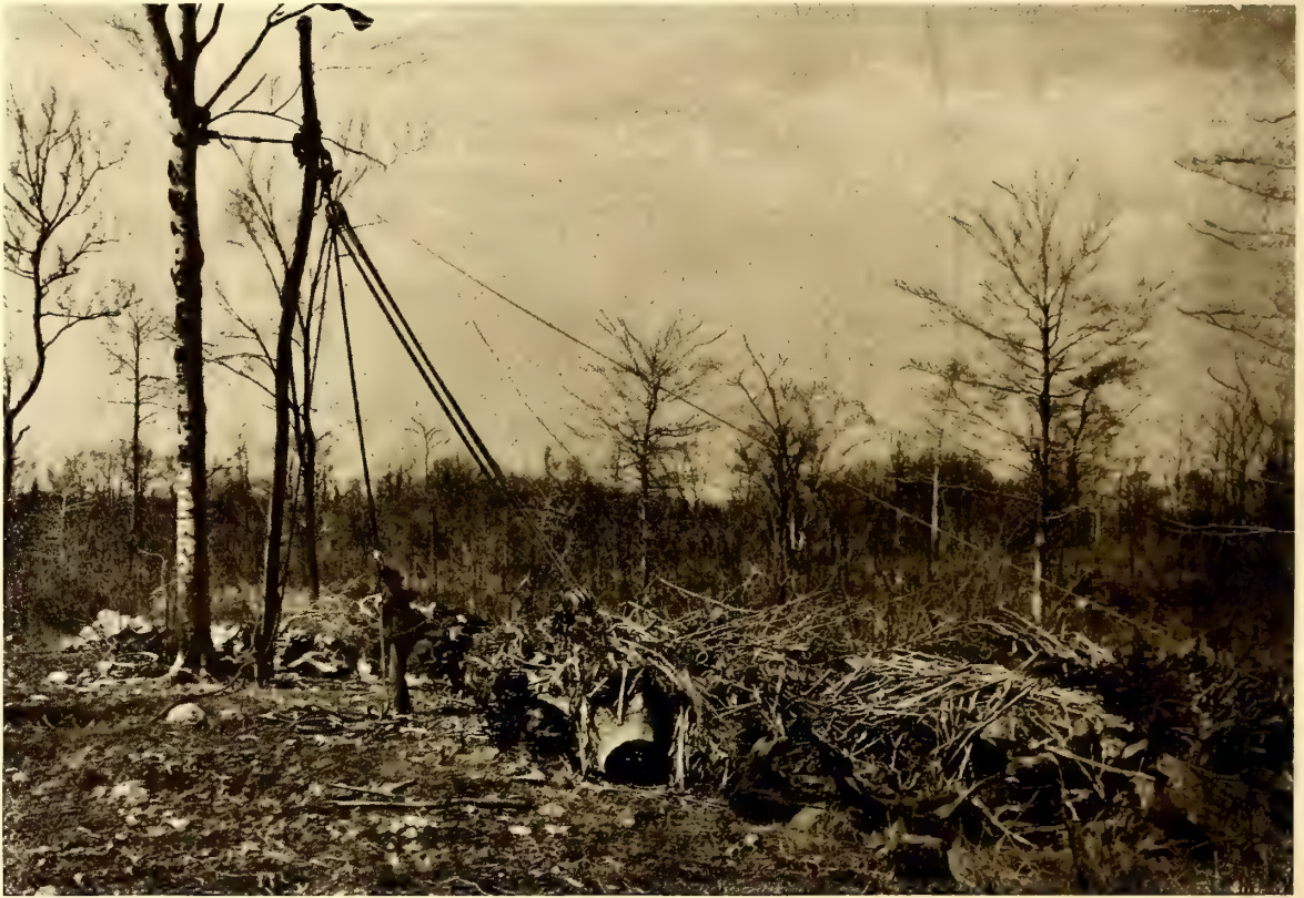
A Pulley Attached to a Tree Is a Convenient Device for Gathering the Stumps and Rubbish for Final Disposal
