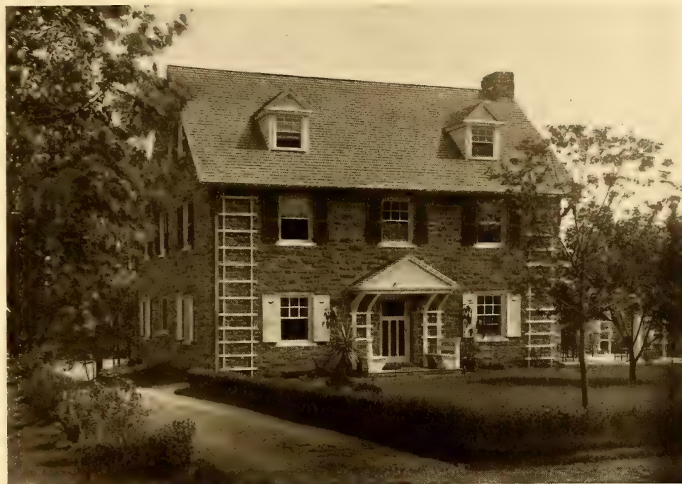
Rock Faced Local Stone Laid in White Mortar with Raked Joints, Is the Material of Which the Exterior Walls Are Built
