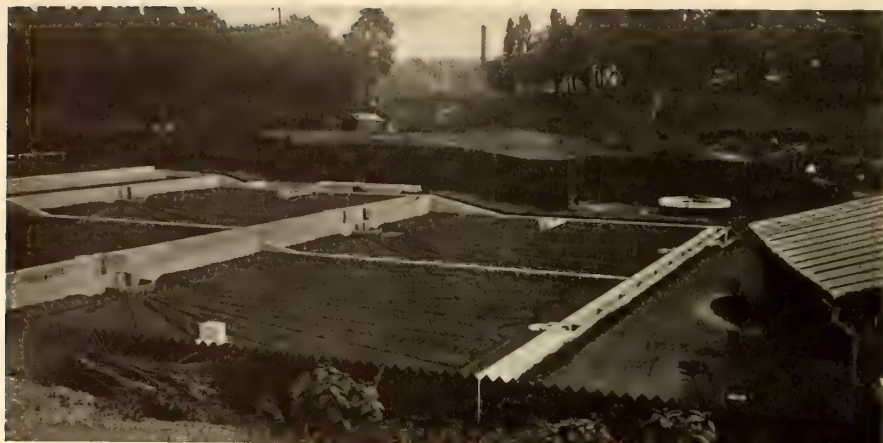
Bacterial Beds of First and Second Contact at La Madeleine-les-Lille
