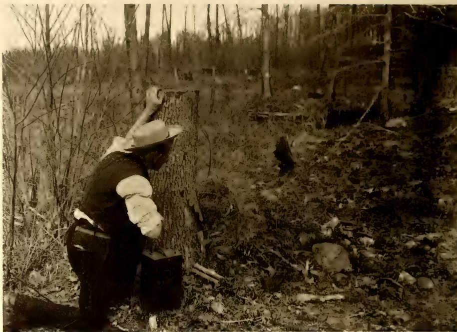
Firing the Dynamite from the Electric Battery
