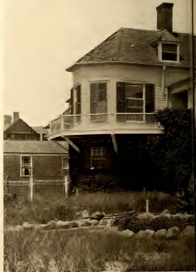
The "Upper Deck" Extends the Living Room and Gives a View of the Ocean
