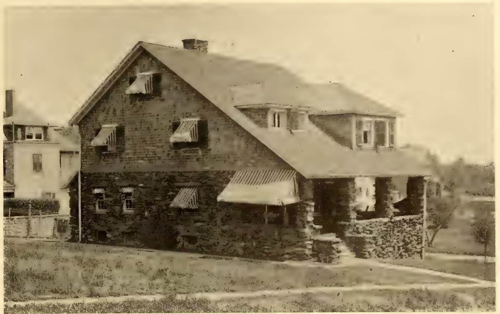
3—Rubble Field Stone and Shingles Are Happily Combined for the Exterior
