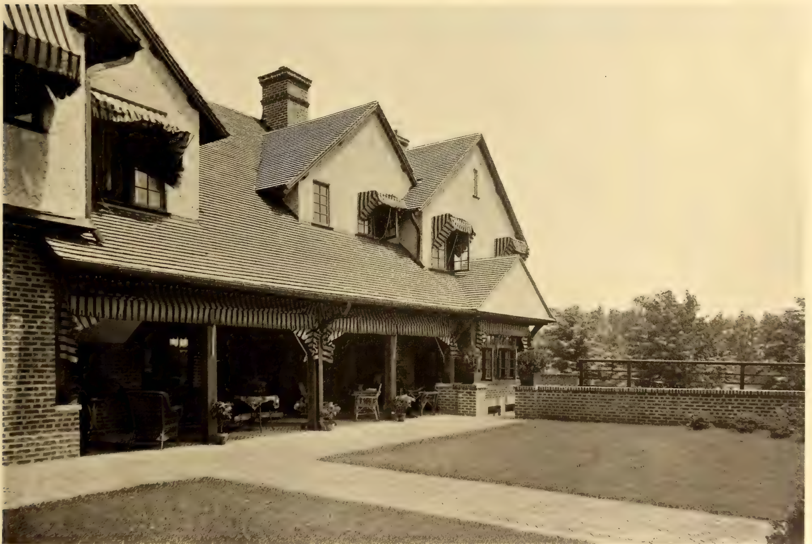
The Loggia Overlooking the Enclosed Terrace
