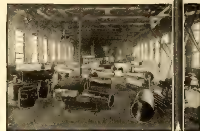
A VIEW IN THE ASSEMBLING ROOM
