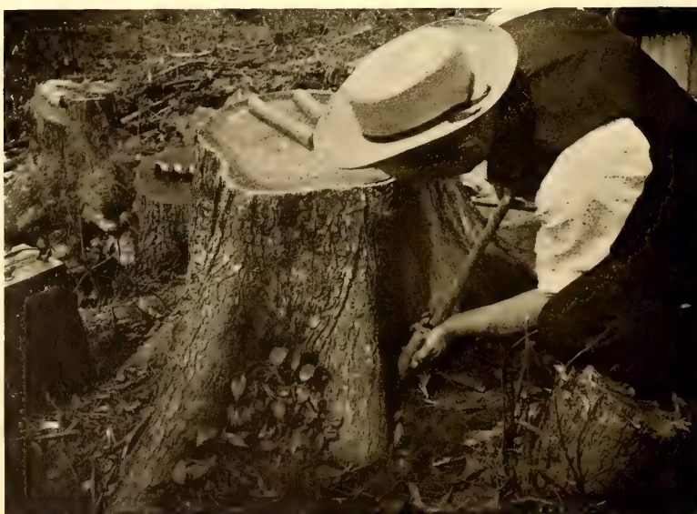
Ramming the Sticks of Dynamite Into Position
