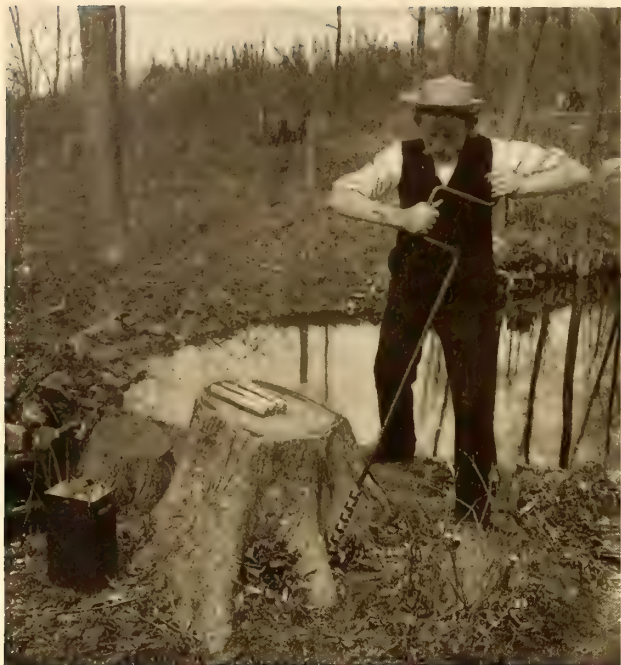
Drilling Auger Holes for the Sticks of Dynamite
