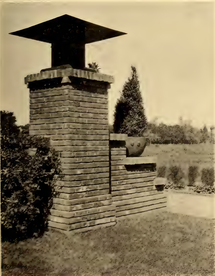
Brick Pier with Japanese Lantern
