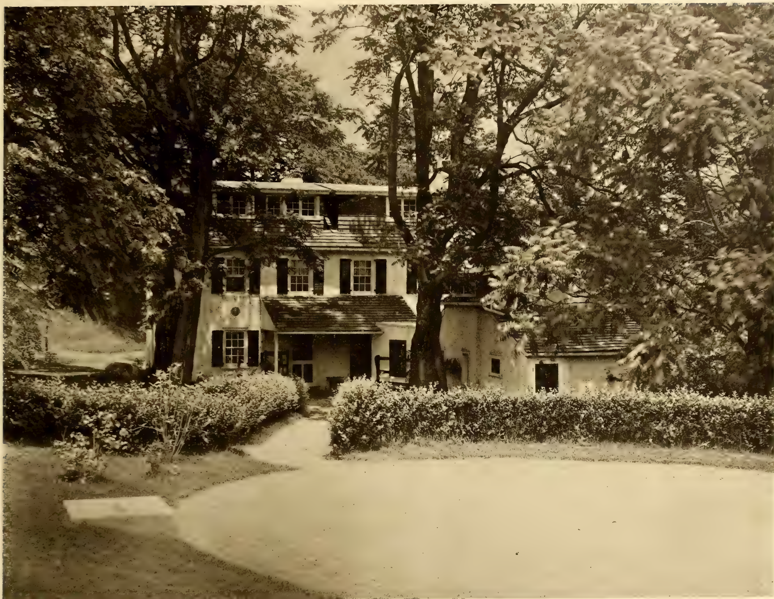
The Old House was Maintained by Plastering the Exterior Walls and Coating Them with Whitewash
