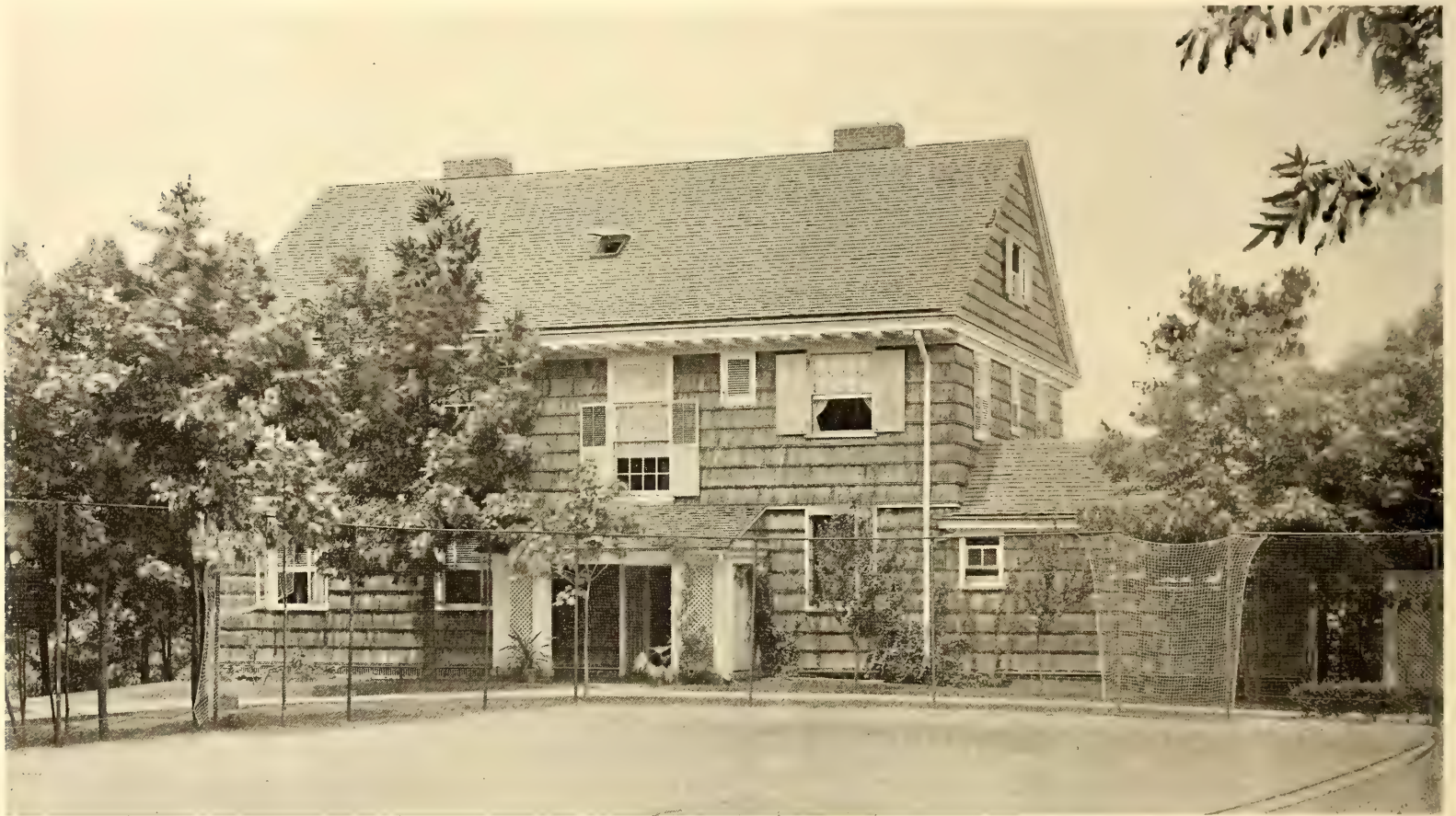
The House Is Covered with Split Shingles
