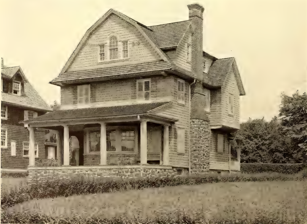
6—Doric Columns Support the Porch Roof
