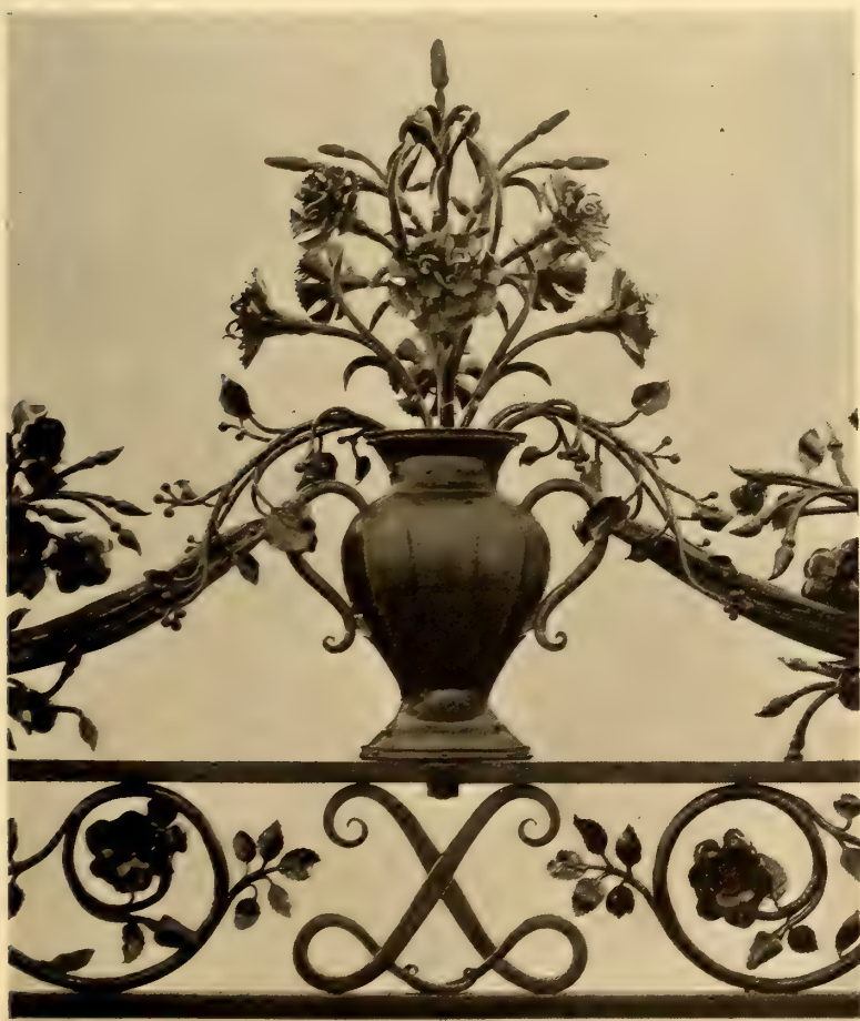
Top Central Section of Gateway Ornamented With Iron Carnations; Each Petal Was Wrought Separately and Then Welded Into Position
