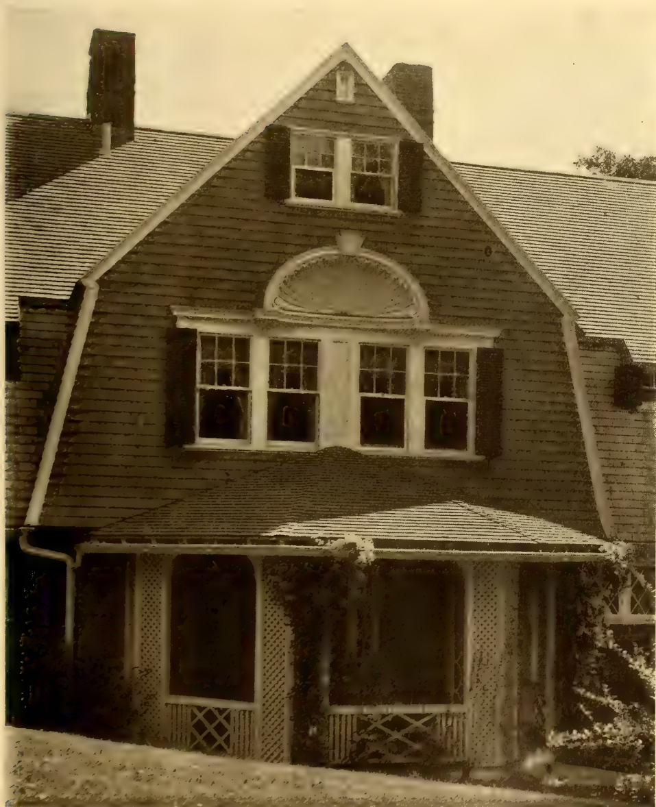
The Entrance Porch Has Latticed Supports
