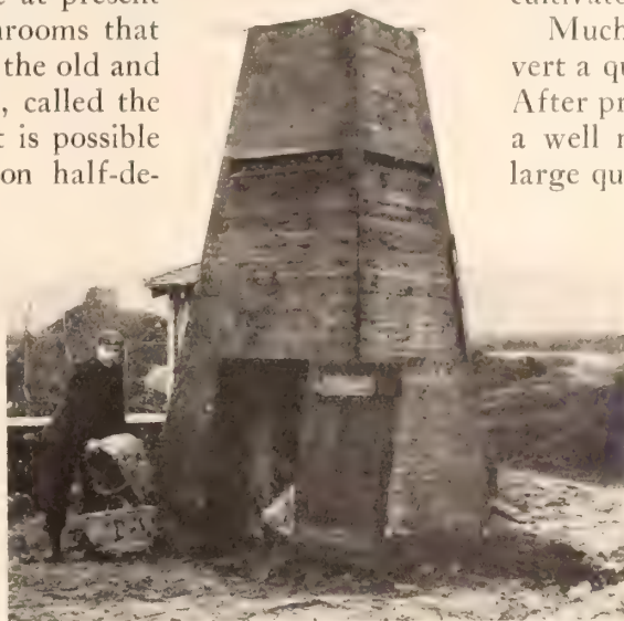
Ventilating-shaft of a Mushroom-cave
