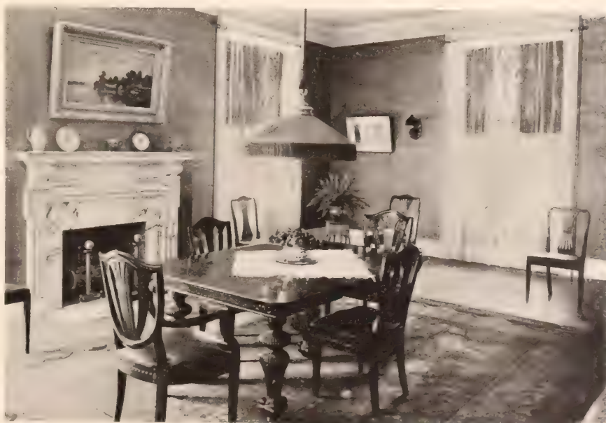
Facings Built of Pavana marble for the Fireplace and a Good Mantel are the Features of the Dining-room
