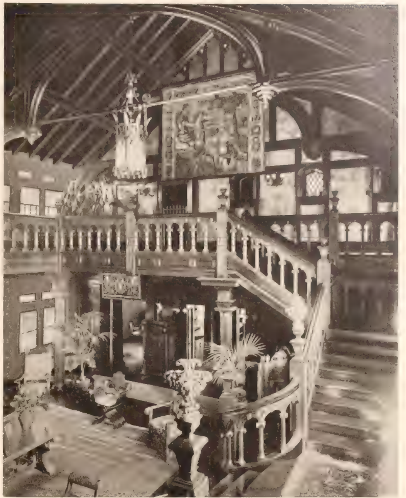
The Hall Has an Open Timber Roof
