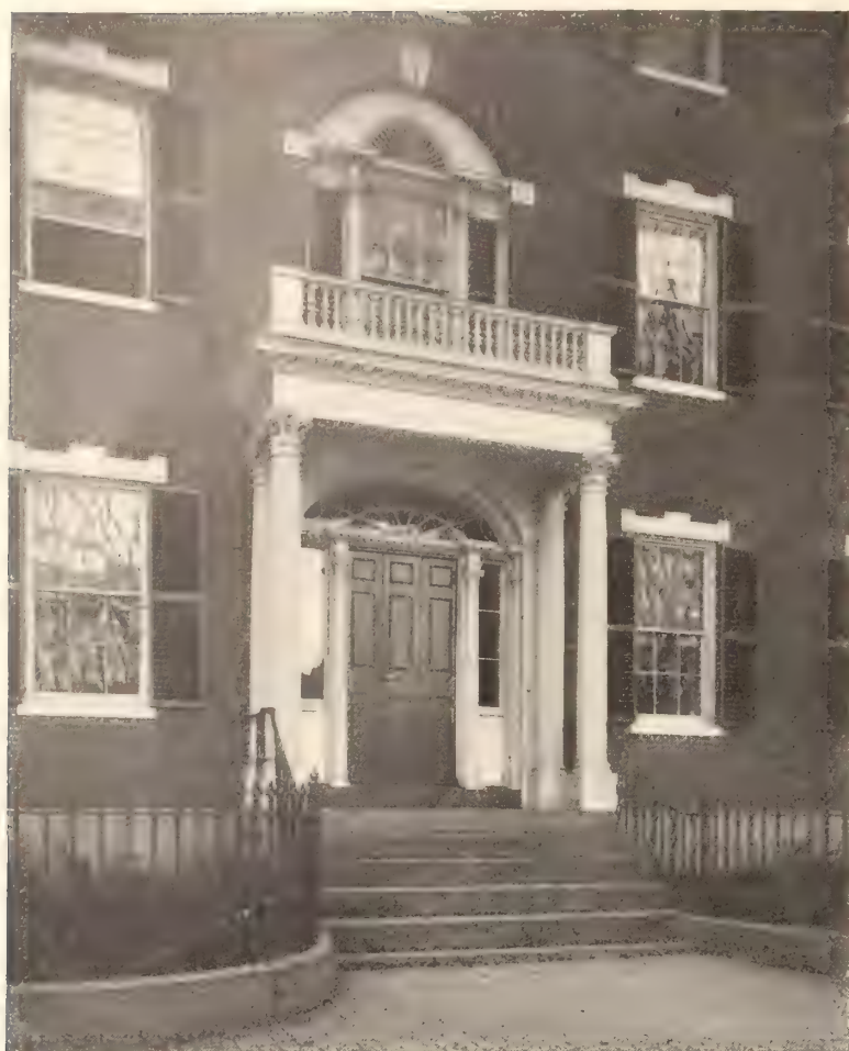
Porch of Dr. Shreve's House
