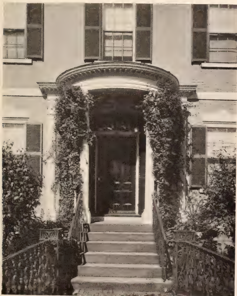
The Porch of Mr. David Pingree's House
