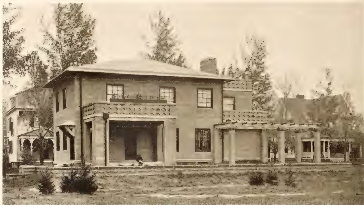
12—House of Mr. W. J. Steel, at New Dorp, Staten Island, is Constructed with Hollow Block Walls and Reinforced Concrete Roof and Floors
