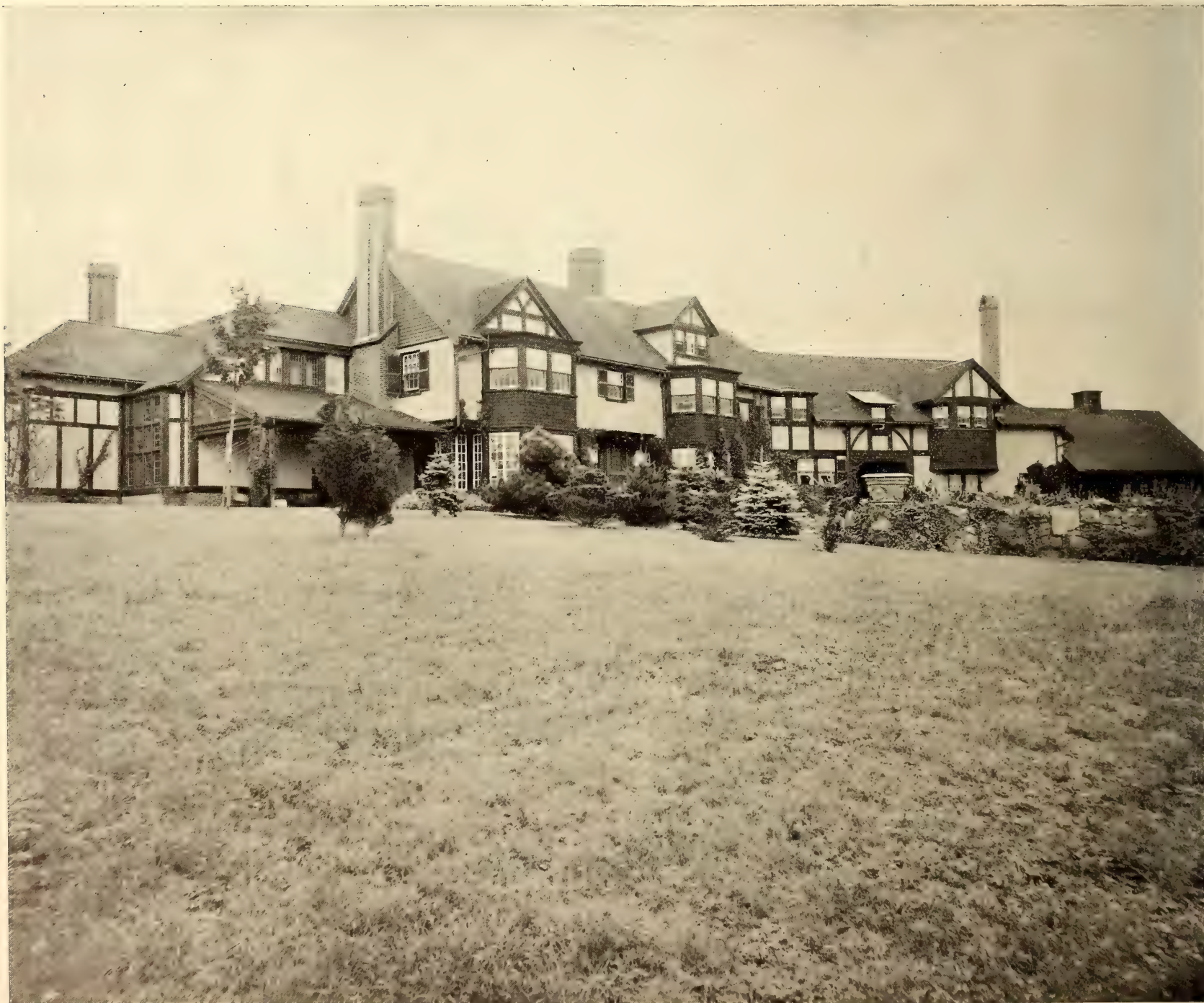
"Craigston"—The Entrance Front
