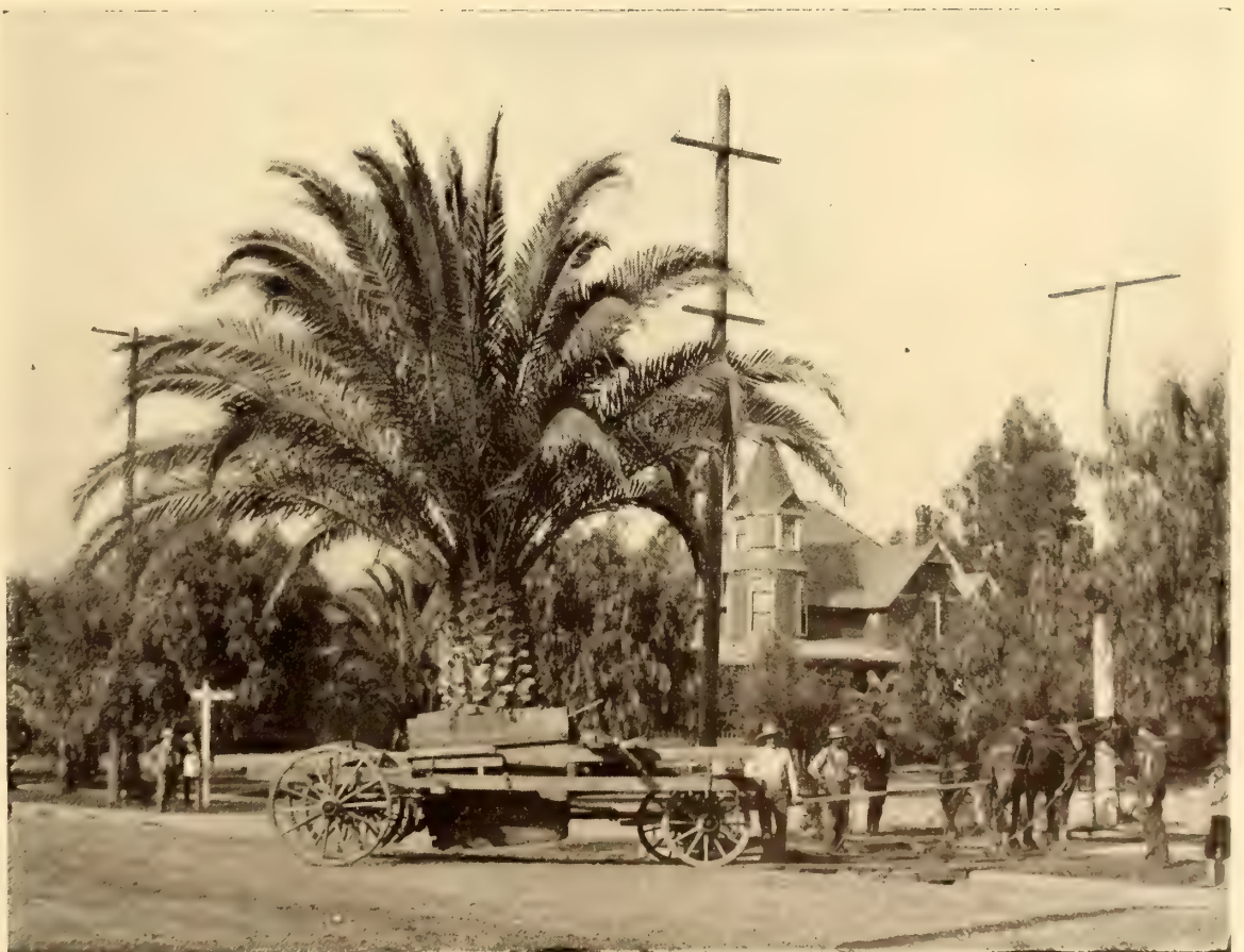
Arrival of the Seven-Ton Date Palm, Showing Box and Method of Suspension
