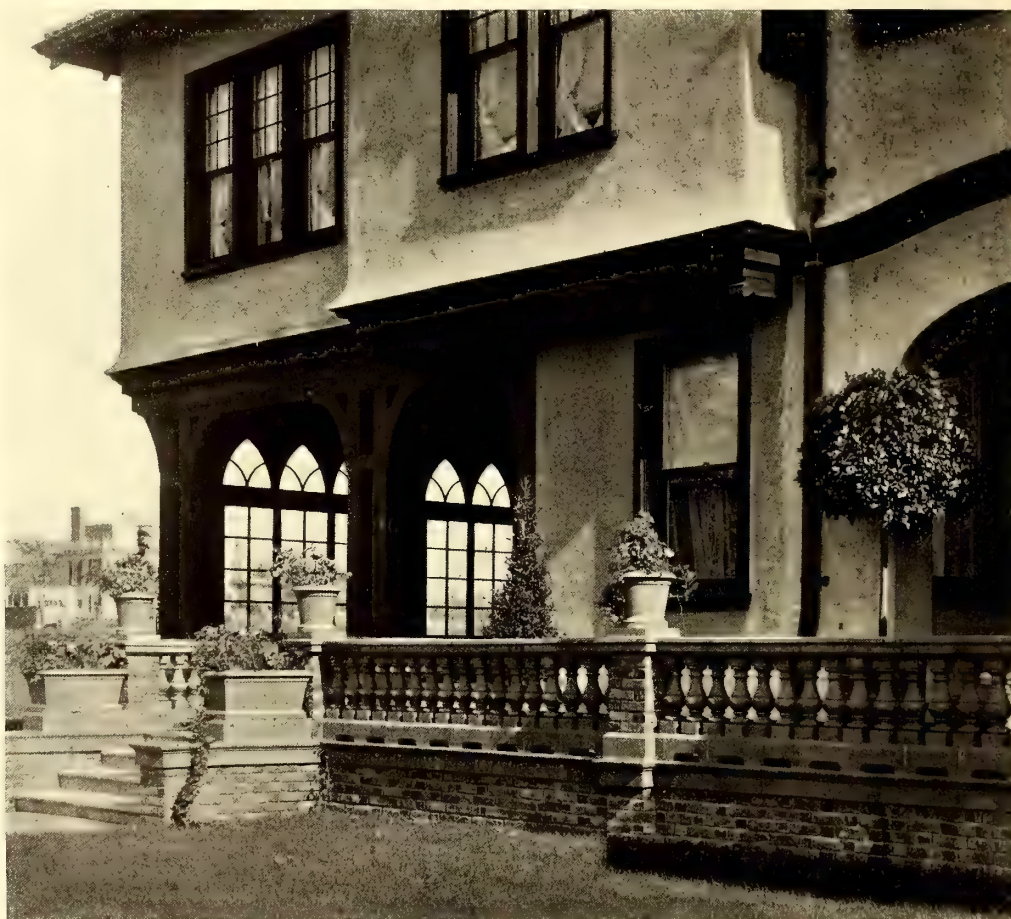
The Entrance Porch and Porte-Cochère
