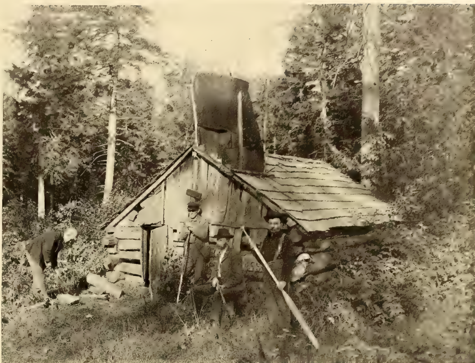
The Use of Boards and Shingles Greatly Simplifies the Work of Construction, But They Are Not Always to Be Obtained
