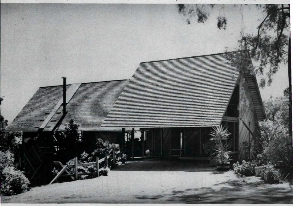
The middle floor of house (above) is on a level with the top of the ravine and is connected to solid land by the drive-way and entry deck. Main wing of house behind carport is supported on stills in middle of the ravine. Concrete piles (right) supporting house have whirled lines left from cardboard pouring forms. The wooden joists, posts, and trusses are left exposed and are incorporated as an important visual element of design.
