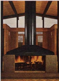
This stalwart fireplace is a freestanding one that divides the living room from the dining room in a California vacation house. The hearth and body are of concrete with exposed aggregate. The metal fire hood and chimney stack are custom made.
