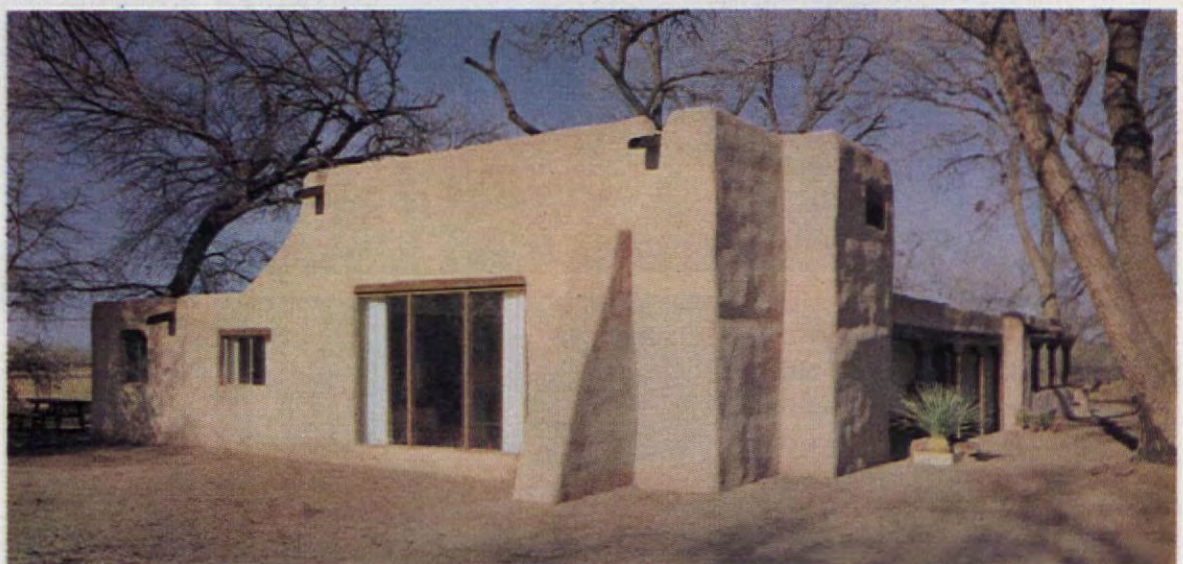
Adobe walls are stucco-covered. Buttress supports the high walls of the living room. Water spouts, or canales , are metal-lined wood. Modern roof was used instead of old type of interlaced branches and adobe.
